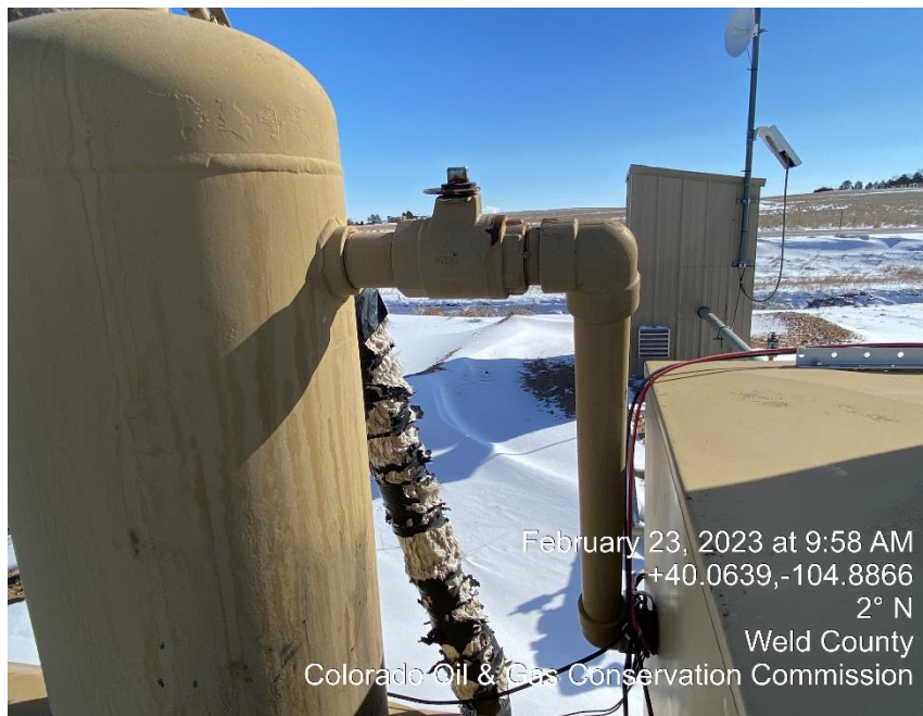
Photo #7 Top-side balloon valve appears to be open
