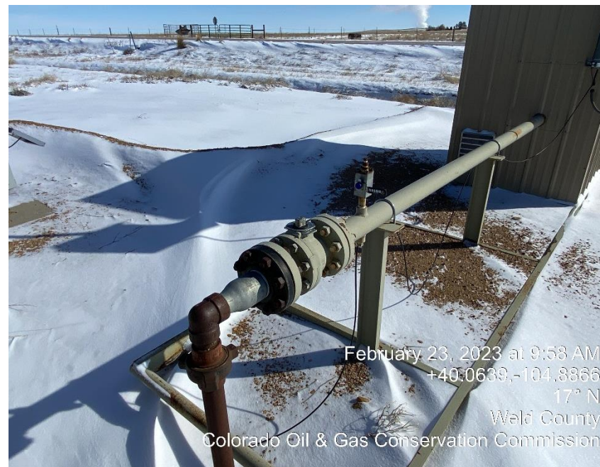
Photo #8 gas meter run balloon on upstream appears open
