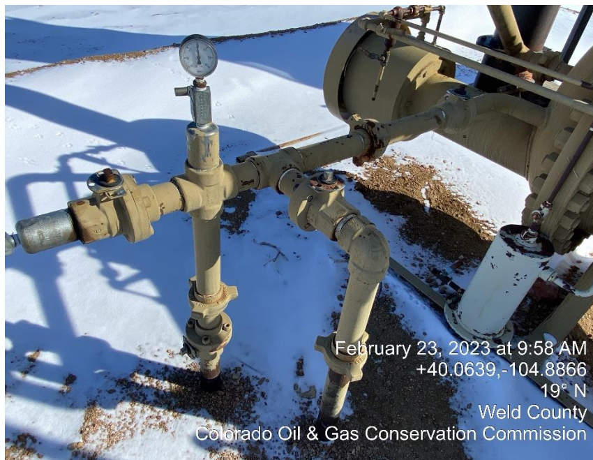
Photo #5 Inlet Balon valve appear to be open
