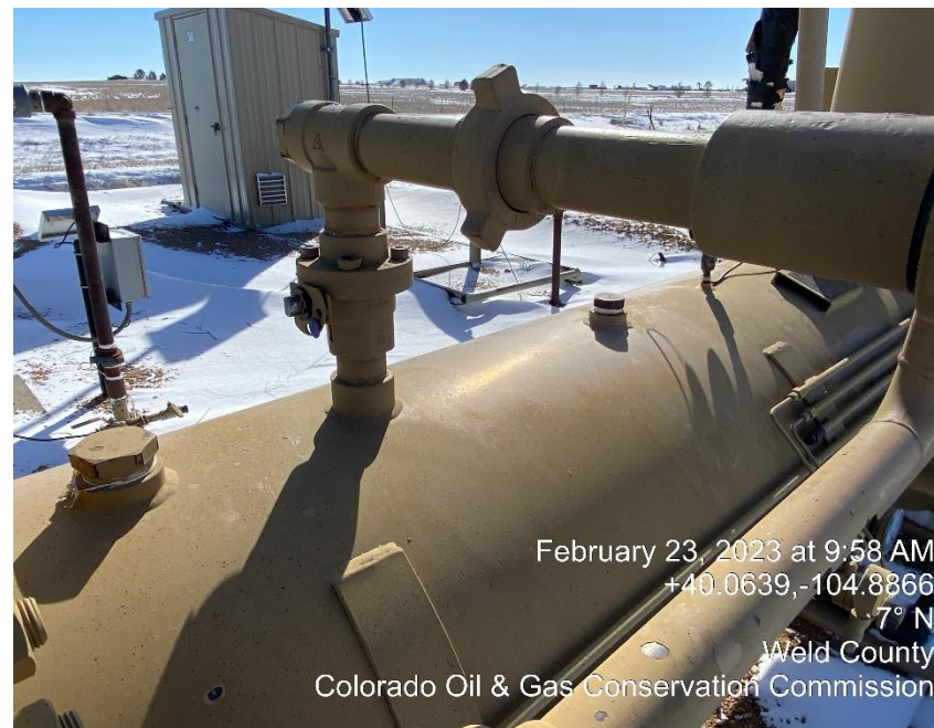
Photo #6 Inlet Balon valve appear to be open
