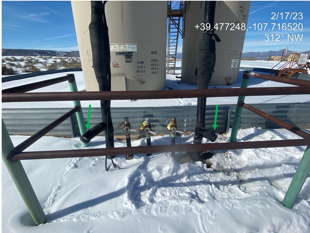
Photo 2. Photo shows caps installed on piping.
