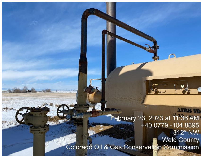
Photo #3 Valves appear to be open
