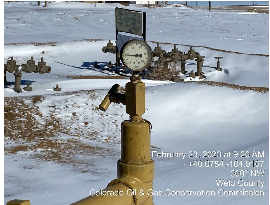
Photo #8 psig appears to so pressure on flowline at the separator
