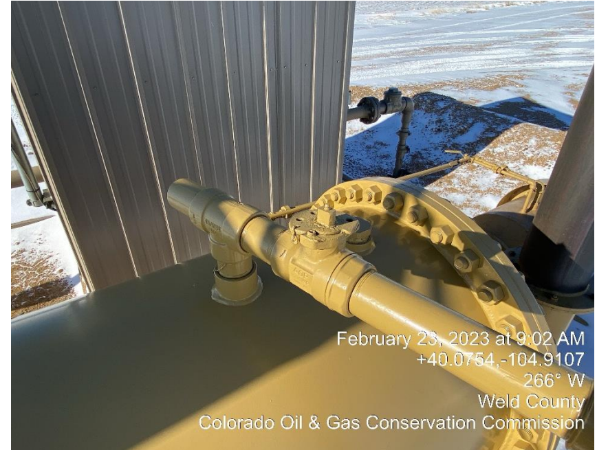
Photo #10 Balon valve appears to be open
