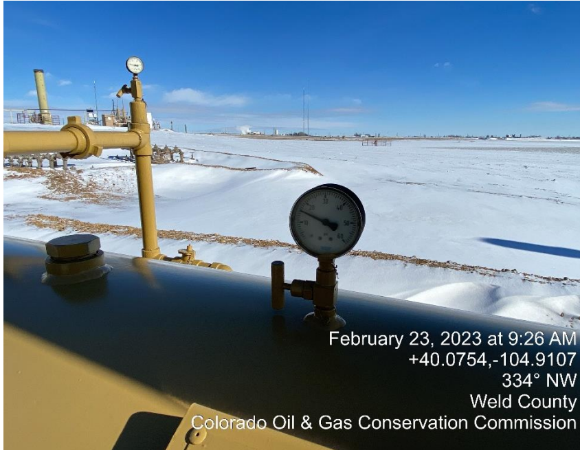
Photo #9 psig appears to show pressure on the separator
