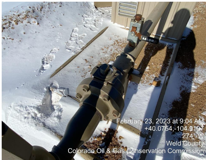
Photo #5 Balon valve on the upstream side appears to be open
