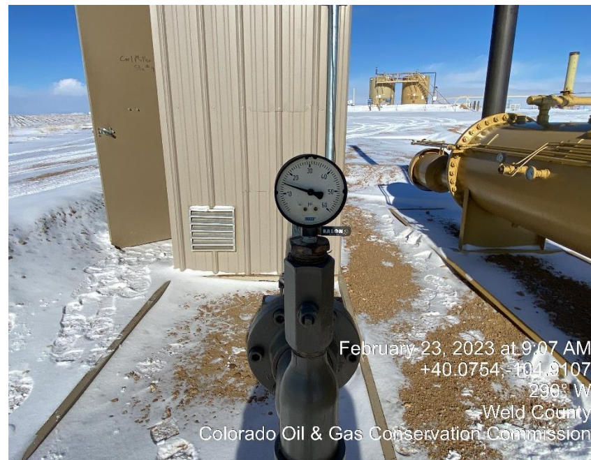
Photo #6 PSI appears to be on the sales gas line from psig
