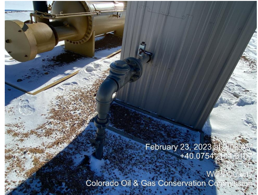
Photo #4 Balon valve on down stream side appears to be open
