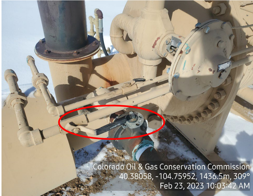
Photo 3: Valves appear to be open
