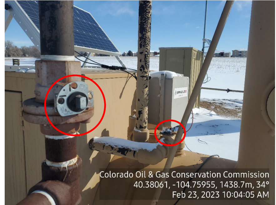
Photo 4: Valves appear to be open
