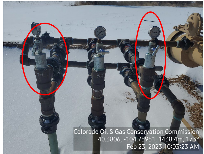
Photo 2: Valves appear to be open
