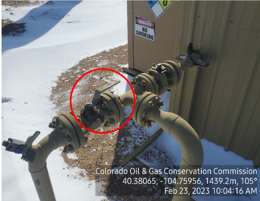
Photo 5: Valve appears to be open
