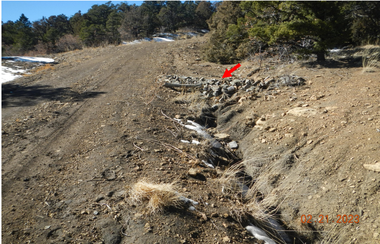
Photo 7. The rock check dam at red arrow is filled in with sediment and there is some erosion below the check dam. Lat/Long:37.15901,-104.99182
