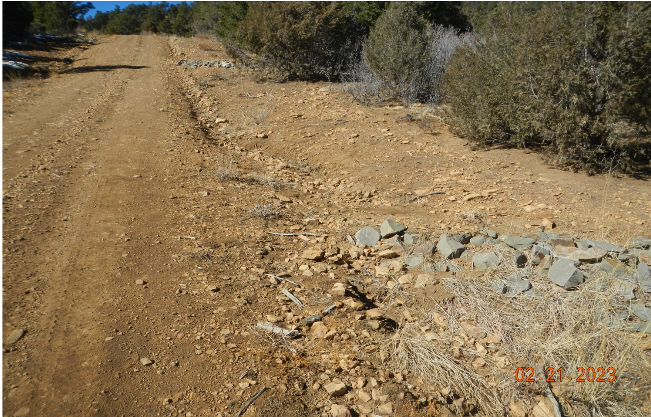
Photo 6. Some of the check dams could use some hand maintenance to allow proper flow away from the roadside.
