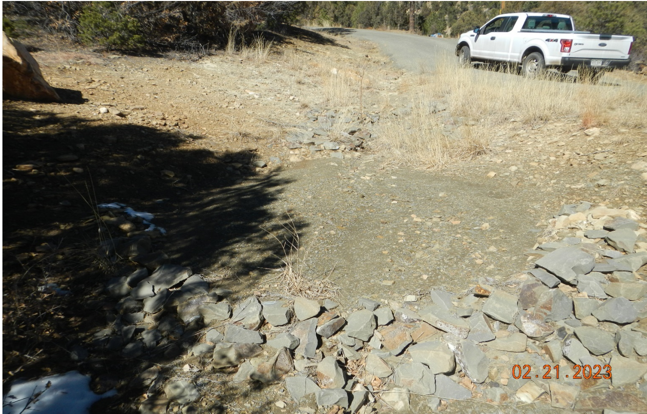
Photo 3. There is sediment accumulation along this rip/rap outlet which needs maintenance (shoveled/cleaned out).
