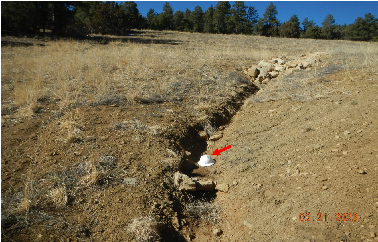
Photo 11. Facing north at the west side of the location. This stormwater diversion is eroding in this area and will need further stabilization. Red arrow points to hard hat for scale.
