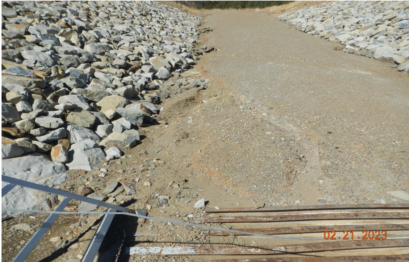
Photo 2. Facing north at the cattleguard. There has been erosion along the road sides and sediment is being deposited into the cattleguard.
