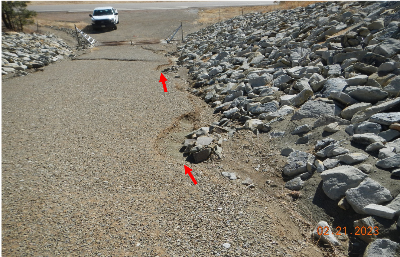
Photo 3. Facing back south on the access road. Sediment has filled in the check dams and stormwater has eroded around the outside shown at red arrows.
