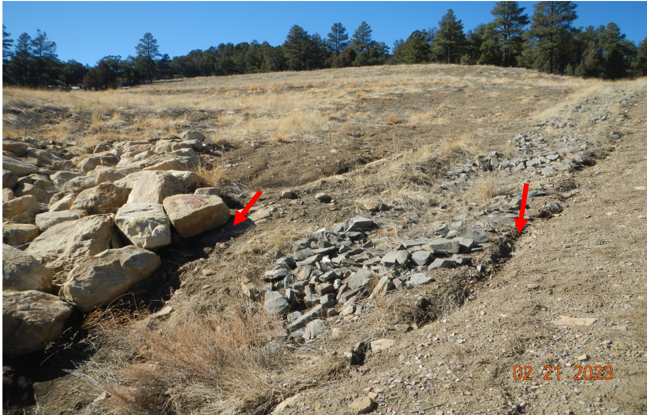
Photo 5. Facing northwest at the recontoured location. It appears stormwater erosion is occurring along the side of the rip/rap which will need maintenance.
