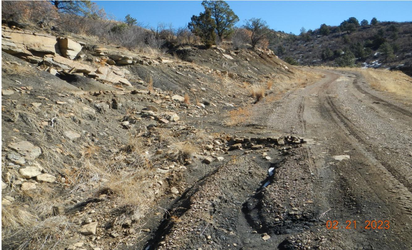
**Photo 2.** Stormwater water which is directed to this area from the wellsite above is causing erosion of the access road in this area.
