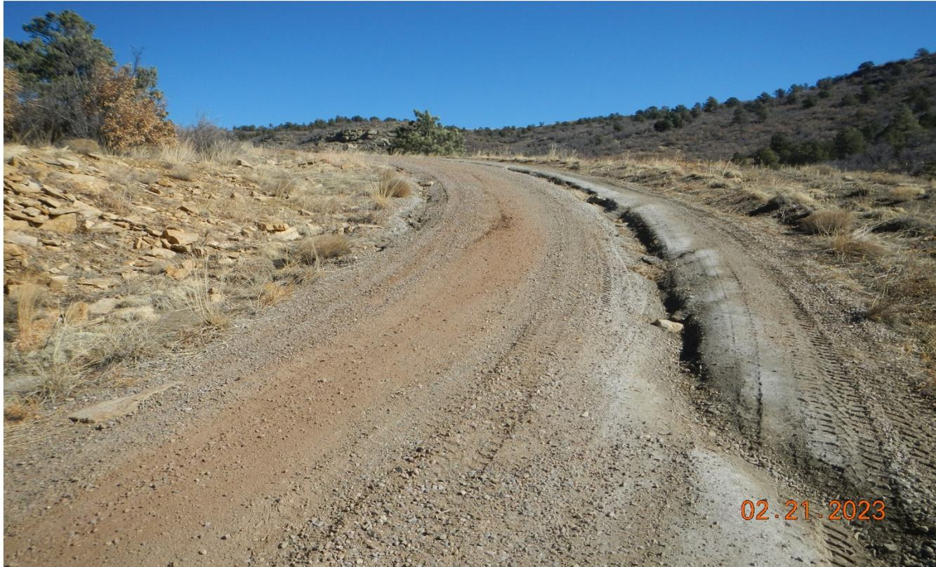
**Photo 3.** There is an erosion channel along the access road ascending to the location.
