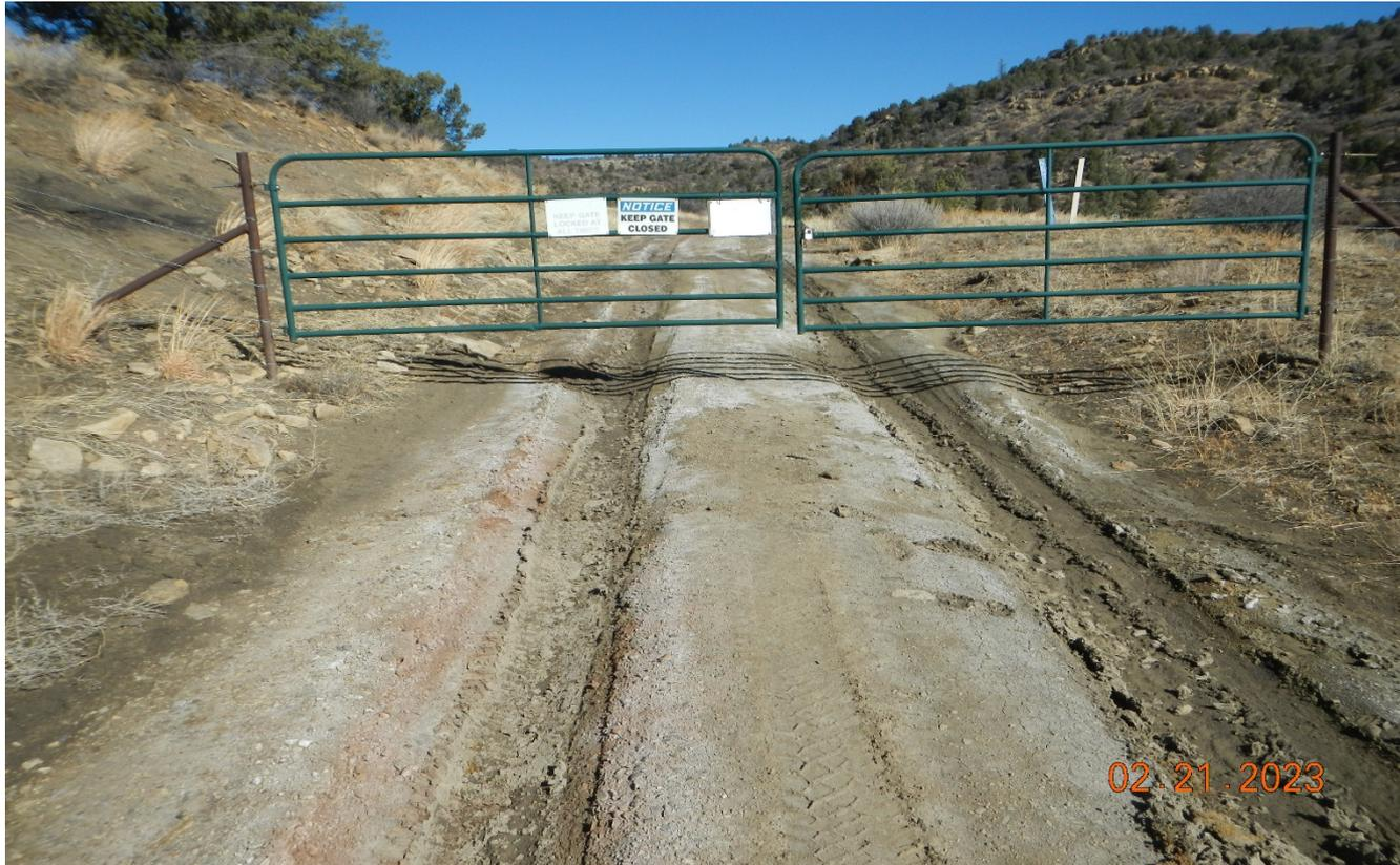
**Photo 1.** Facing north along the access road which is rutted and eroded in this area.
