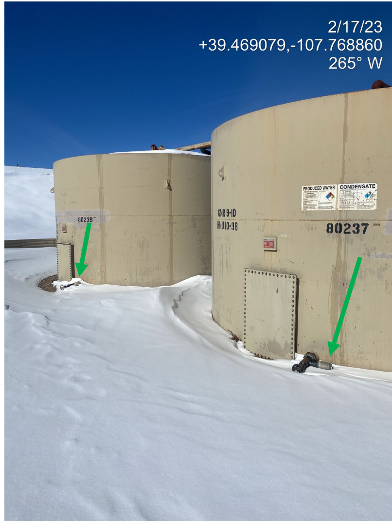
Photo 2. Photo shows drain line bull plugs installed.
