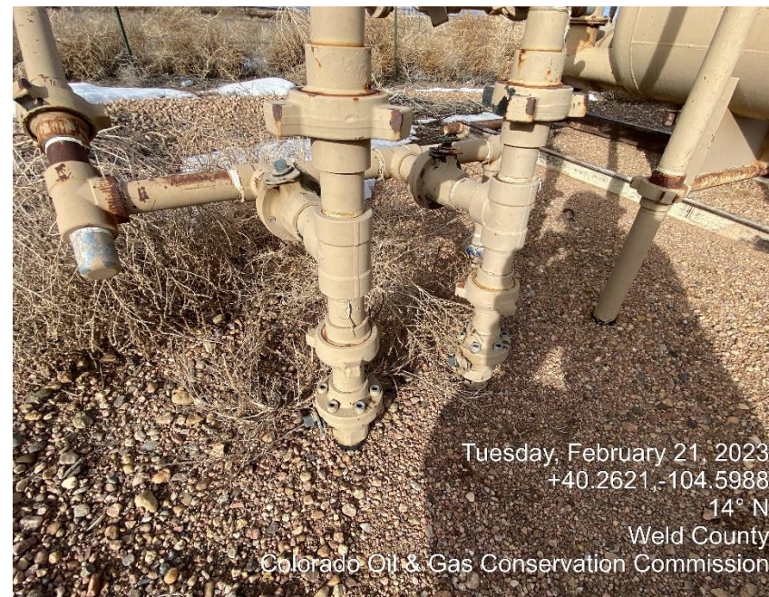
Photo #4 Balon valves appear open at the headed at the separator
