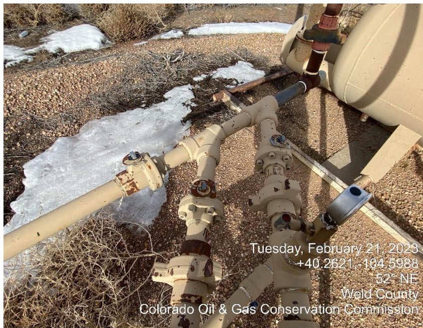
Photo #5 Balon valves at the separator appear to be open
