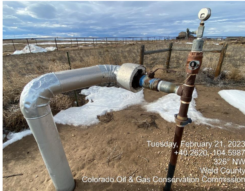
Photo #7 Riser for sales gas appears to be open
