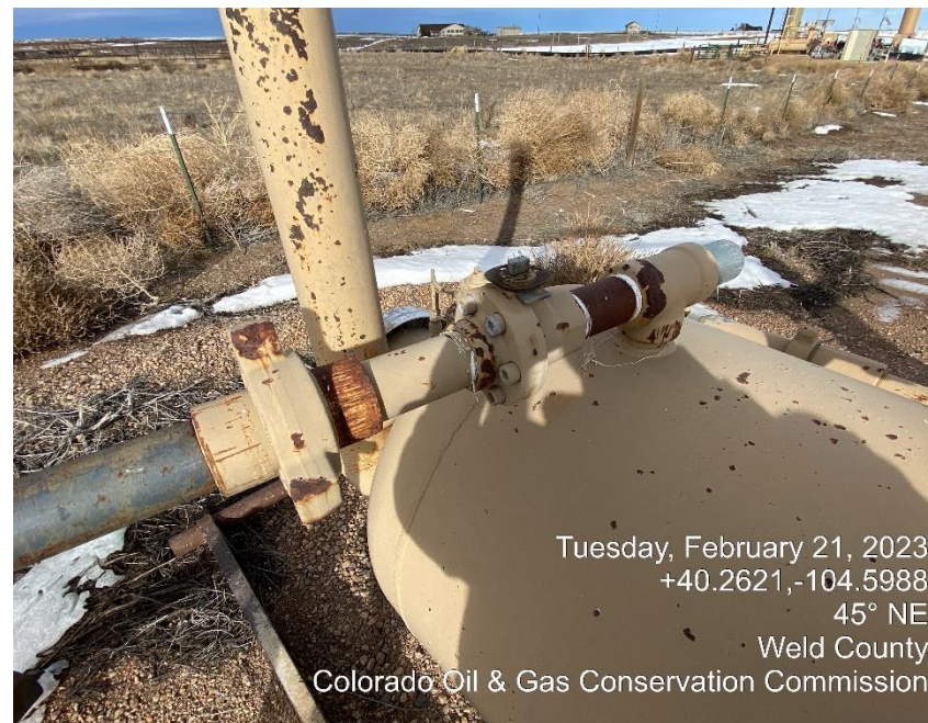
Photo #6 Balon valve appears open going into the separator
