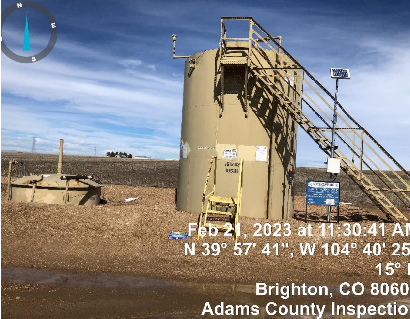
Photo#1 Production Tank and Produced Water tank
