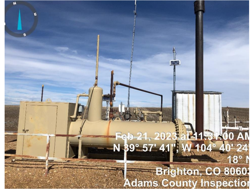
Photo#2 Separator/Gas Meter/Automation RTU
