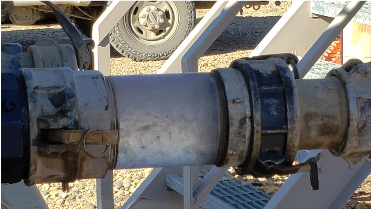
Figure 3 - Transparent Pipe Spool at Suction Truck Showing Clear Water After Flushing
