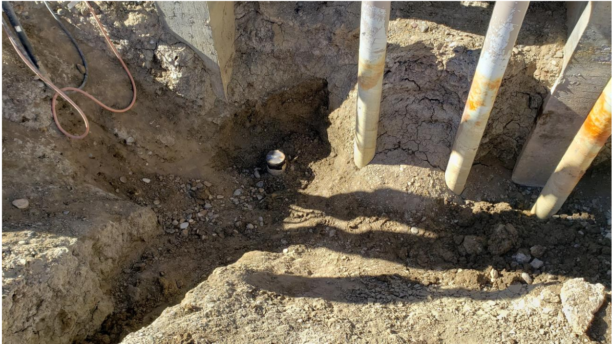
Figure 5 - Capped Flowline at Satellite 38 Header End
