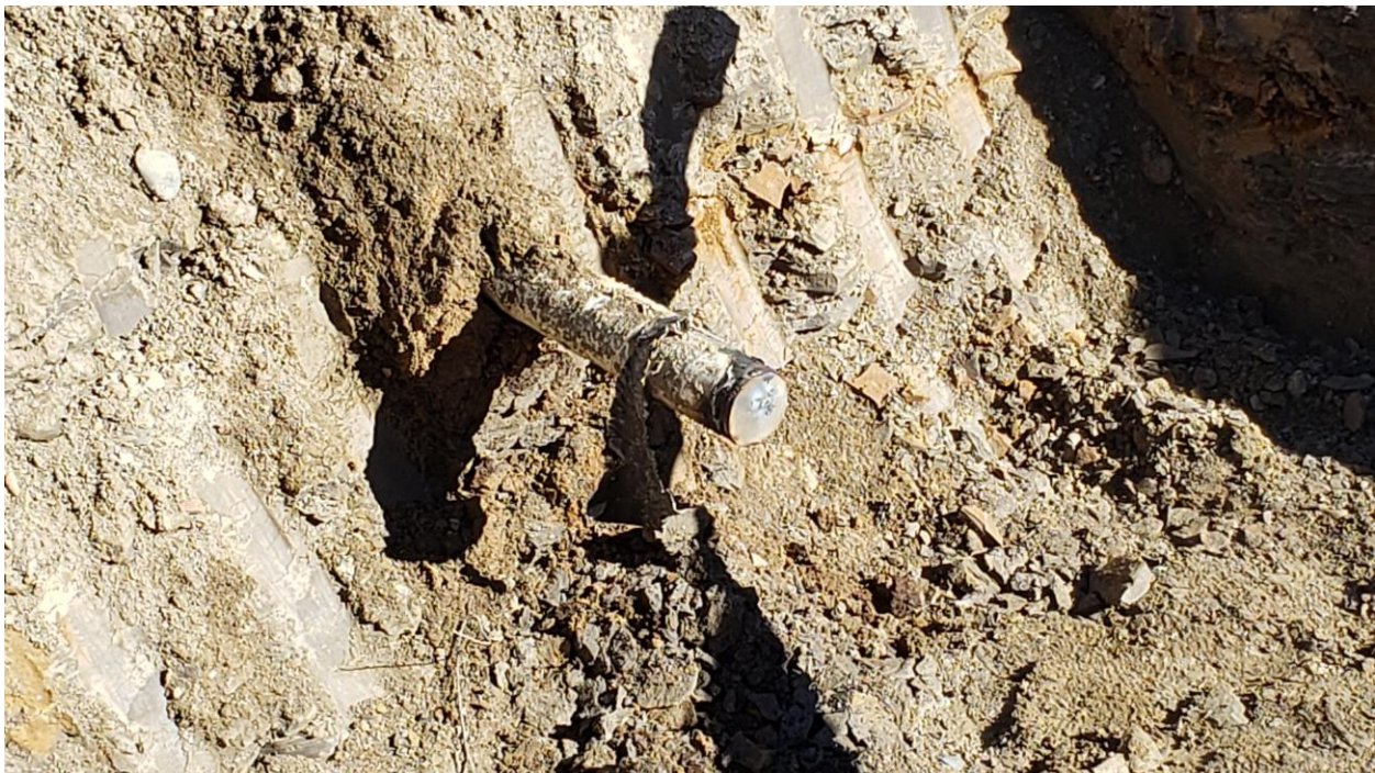
Figure 4 - Capped Flowline at M. B. Larson C11X25 End.
