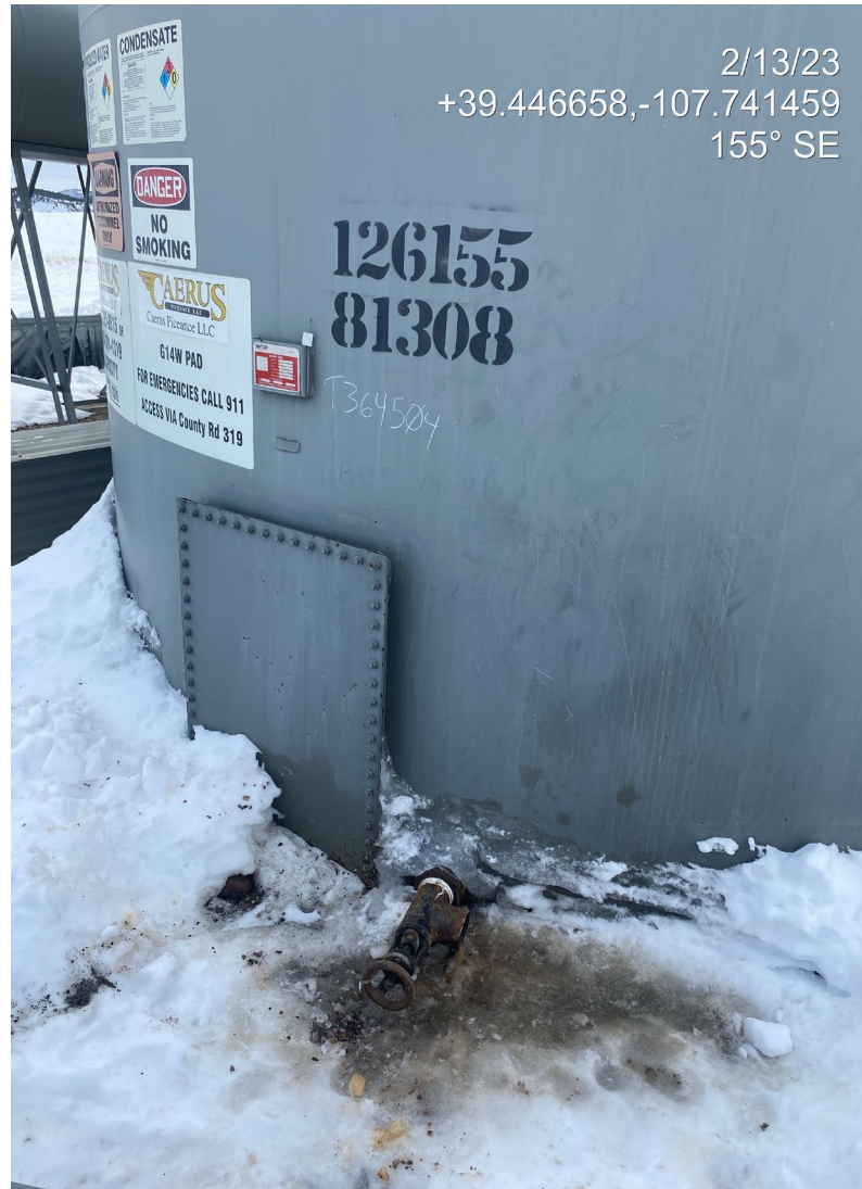
Photo 1. Photo shows a tank drain is not bullplugged.
