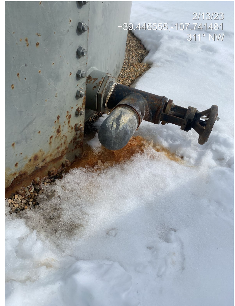
Photo 2. Photos show staining below a produced water/condensate tank drain.
