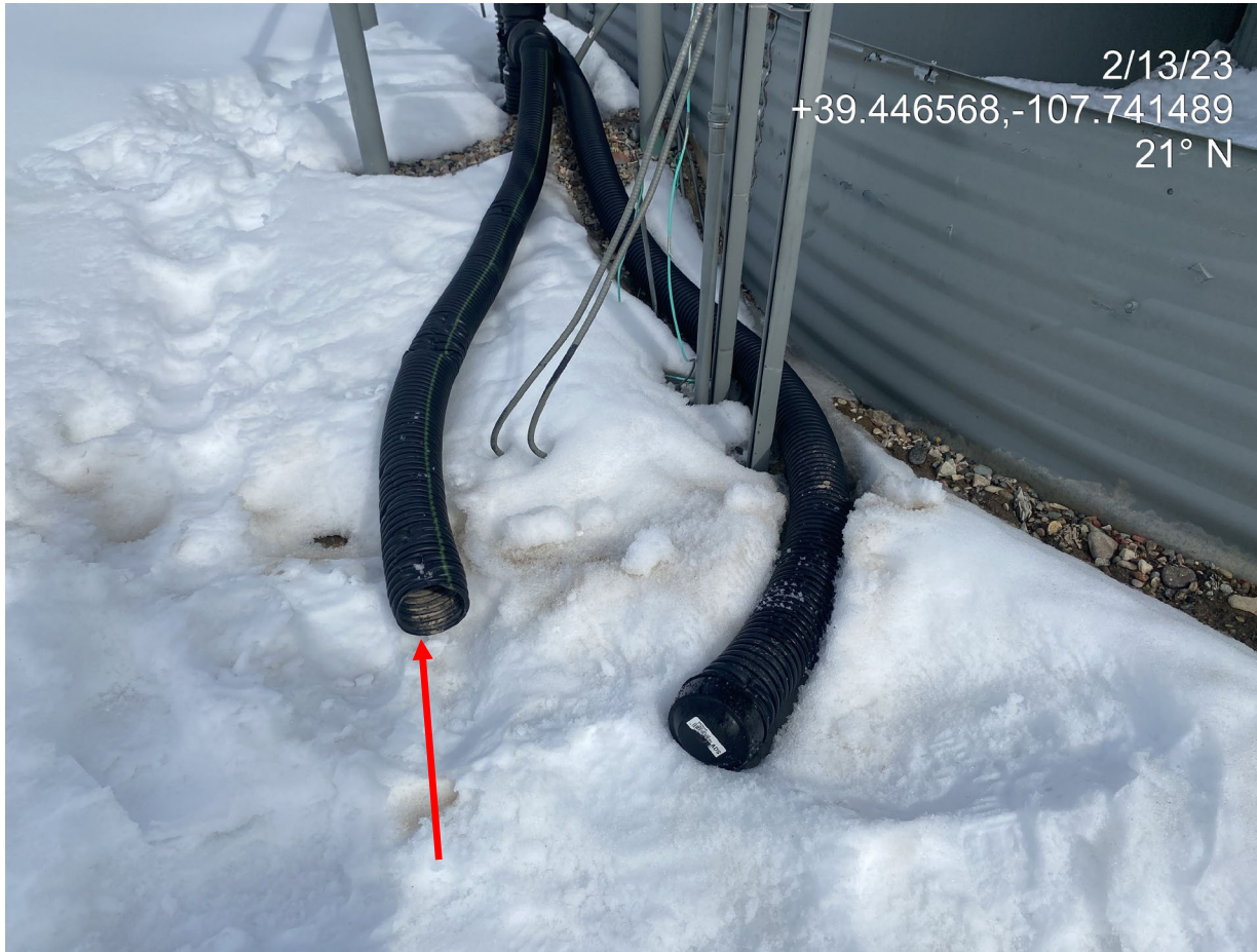
Photo 3. Photo shows piping at the tank battery is open ended and lacks BMPs to prevent wildlife entry.
