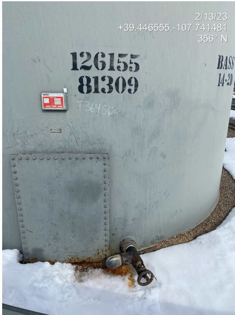
Photo 2. Photos show staining below a produced water/condensate tank drain.
