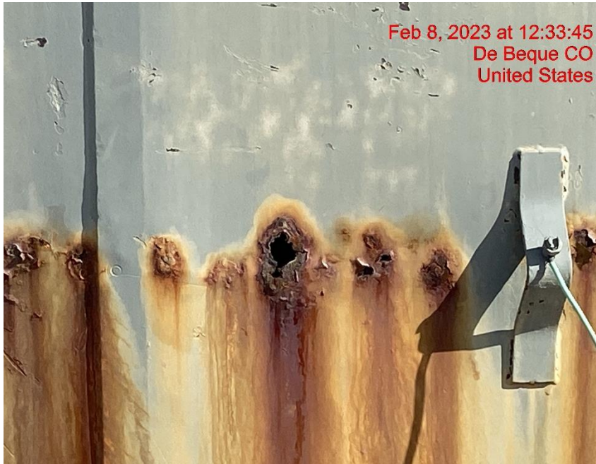
Hole in Tank Wall – Photo #00755
