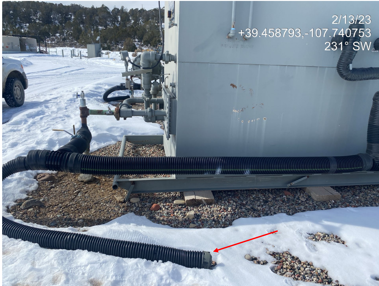
Photo 2. Photo shows a cap has been installed on separator piping per previous corrective action.
