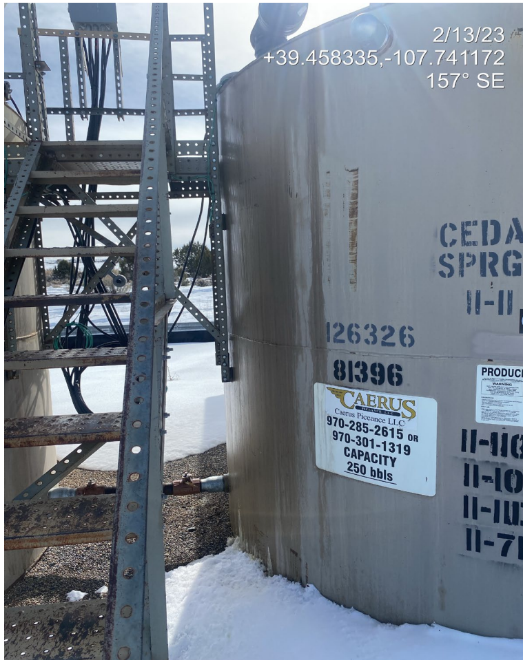
Photo 1. Photos show produced water/condensate tank # 81396 appears to have spilled from the top. Stained gravel observed in secondary containment below the spill (right).
