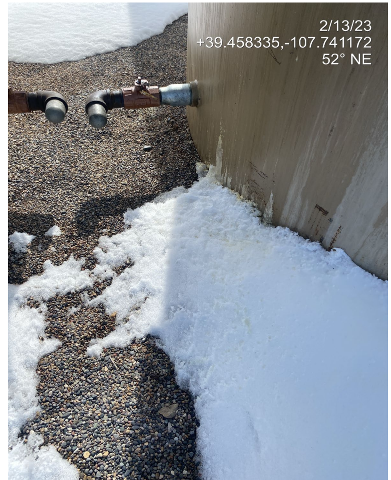
Photo 1. Photos show produced water/condensate tank # 81396 appears to have spilled from the top. Stained gravel observed in secondary containment below the spill (right).
