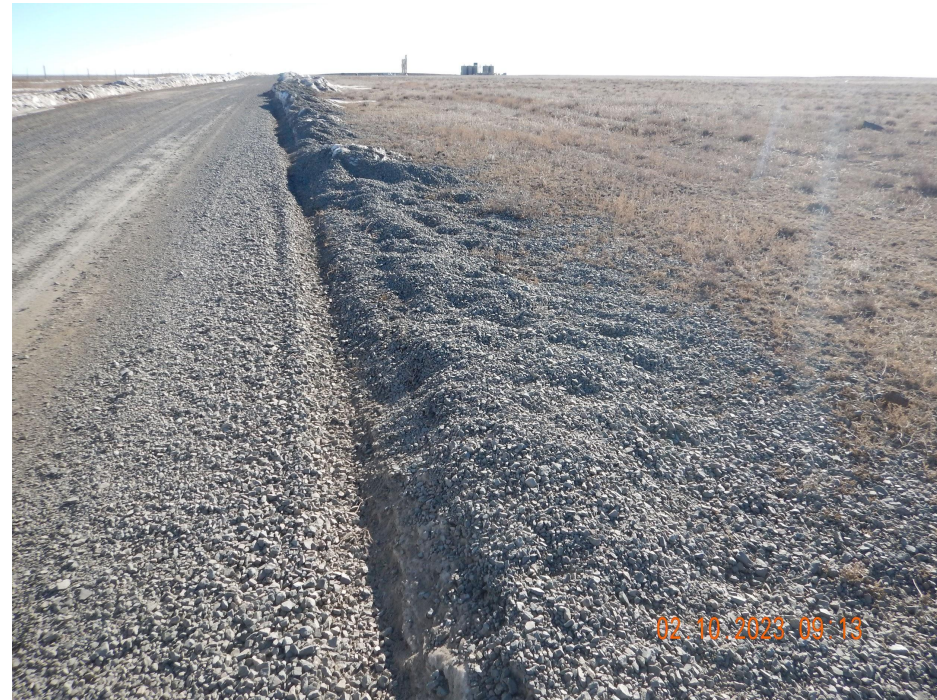
Photo 10. Photo taken from a portion of the access road, facing East. Photo illustrates Operator has conducted snow removal on the access road and is creating additional disturbances by plowing road base onto reference areas.
