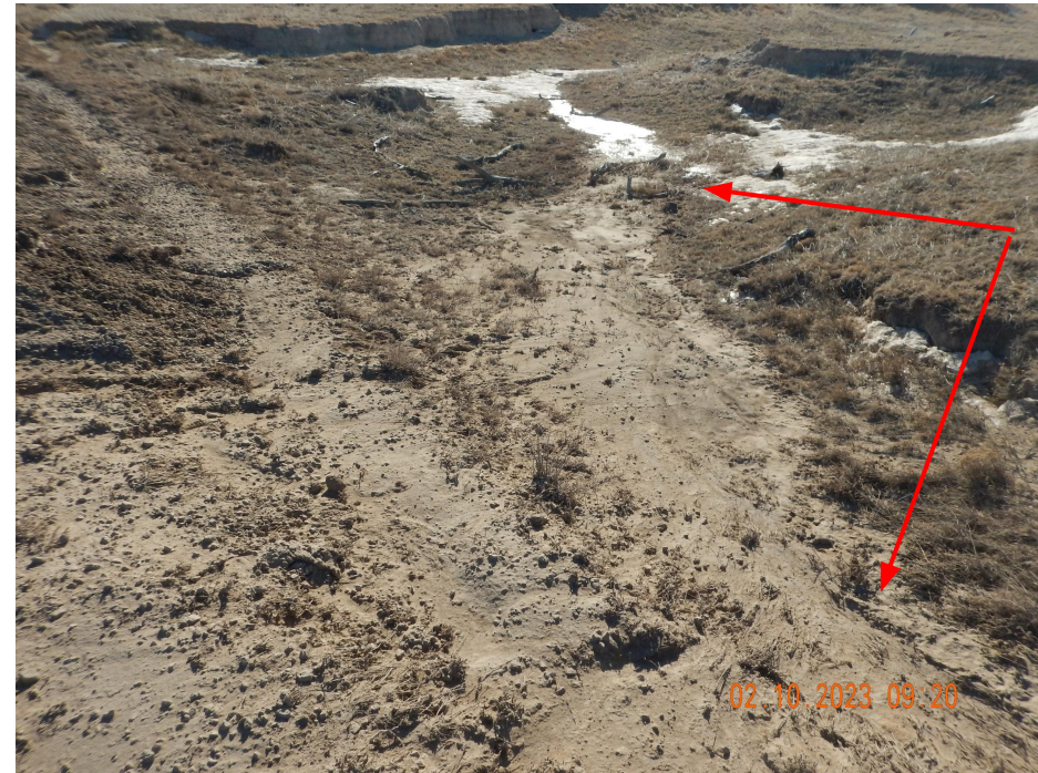
Photo 6. Photo taken from Geary Creek, facing South. Photo illustrates sediment discharge into Geary Creek.
