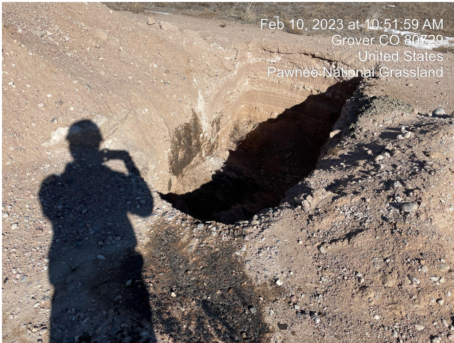
Photo 19. Photo taken from the northeastern location. Photo illustrates an excavation approximately 3'x 8' in size with an unknown depth but ~5-6' deep, which would be considered a pit. The western sidewall of the excavation had observed soil staining, as well as the surface adjacent to the excavation. Also, there is no wildlife fencing or netting.
