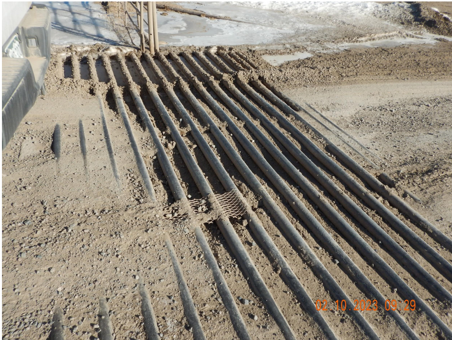
Photo 9. Photo taken from a portion of the access road, facing North. Photo illustrates the cattle guard is not in proper functioning condition to exclude cattle.
