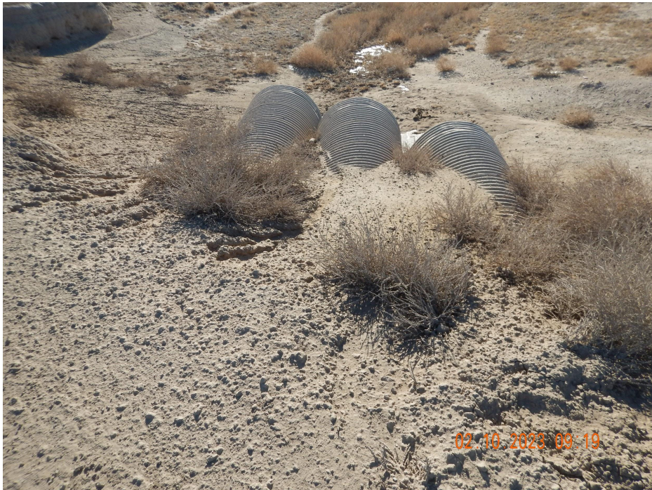
Photo 7. Photo taken from intersection of the access road and Geary Creek, facing South. Photo illustrates sediment discharge into Geary Creek without stormwater BMPs.
