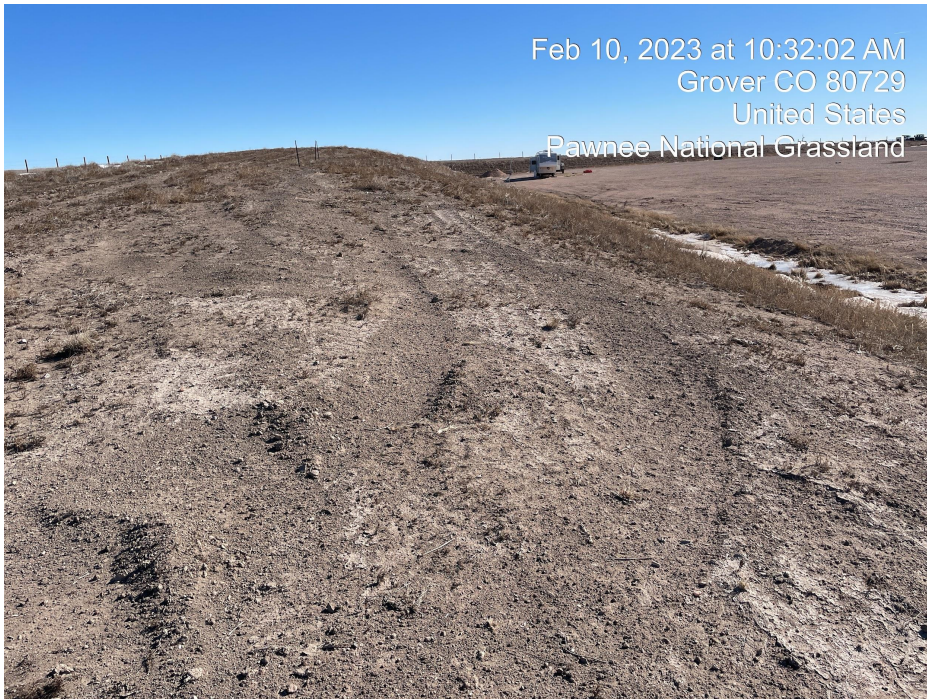
Photo 21. Photo taken from the northwestern location, facing East. Photo illustrates the topsoil stockpile which is bare or has weedy, annual vegetation.
