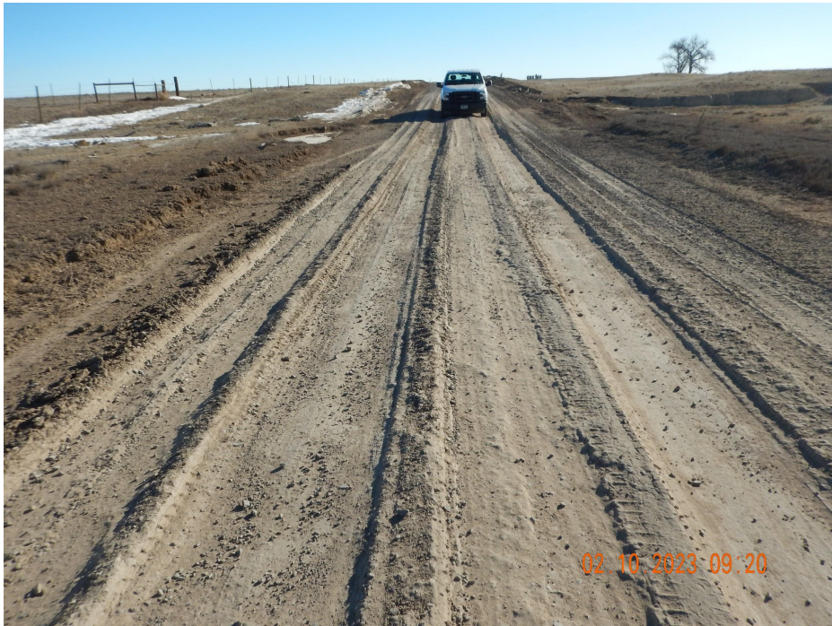
Photo 5. Photo taken from the intersection of the access road and Geary Creek, facing East. Photo illustrates the access road is not sufficiently stabilized which is contributing to sediment discharge into Geary Creek.
