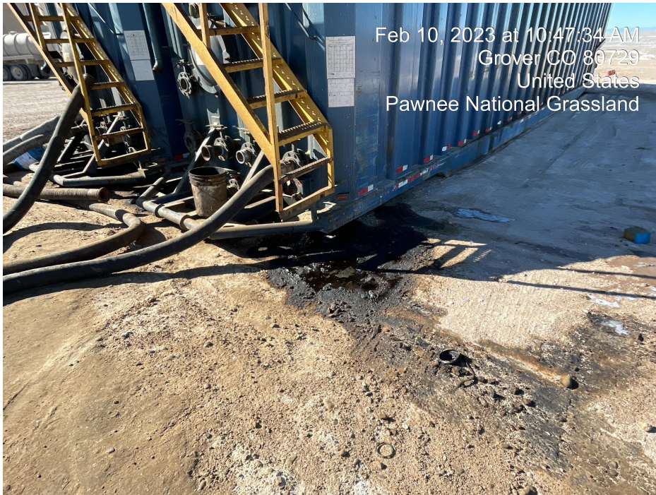
Photo 17. Photo taken from a frac tank on location. Photo illustrates frac tank is leaking oily waste. Oily waste appears to be underneath the frac tank.
