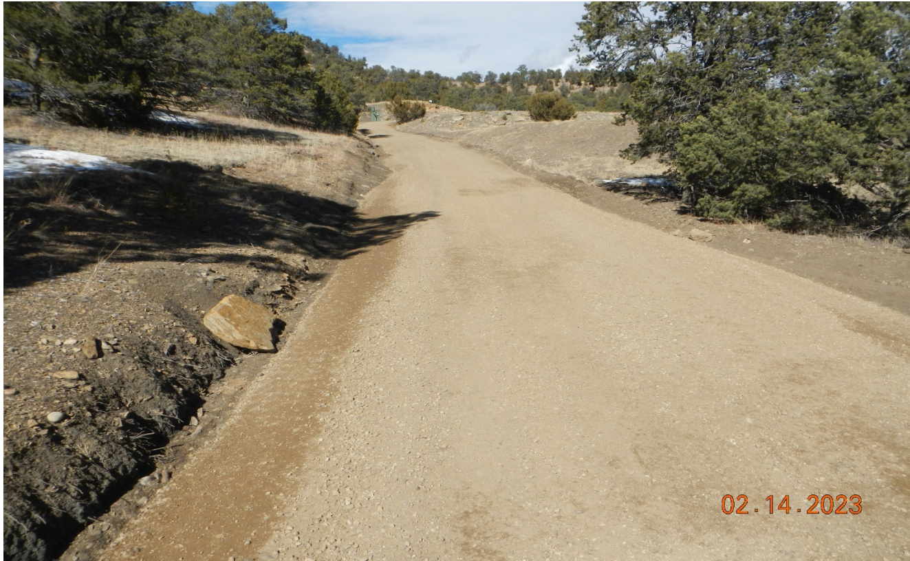
Photo 2. Facing north along the access road. The roadside which was eroded has been repaired but there is no BMP's to prevent erosion from reoccurring (e.g. check dams, riprap, culvert ect).
