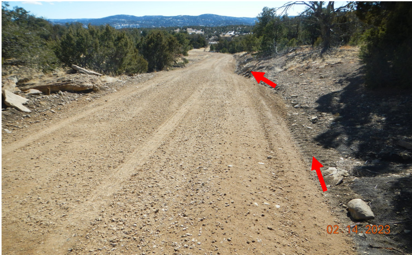
Photo 3. Facing back south toward the access road. This long stretch of road has no roadside BMPs to prevent erosion from reoccurring. Red arrow points to stormwater flow which will occur down the roadside.
