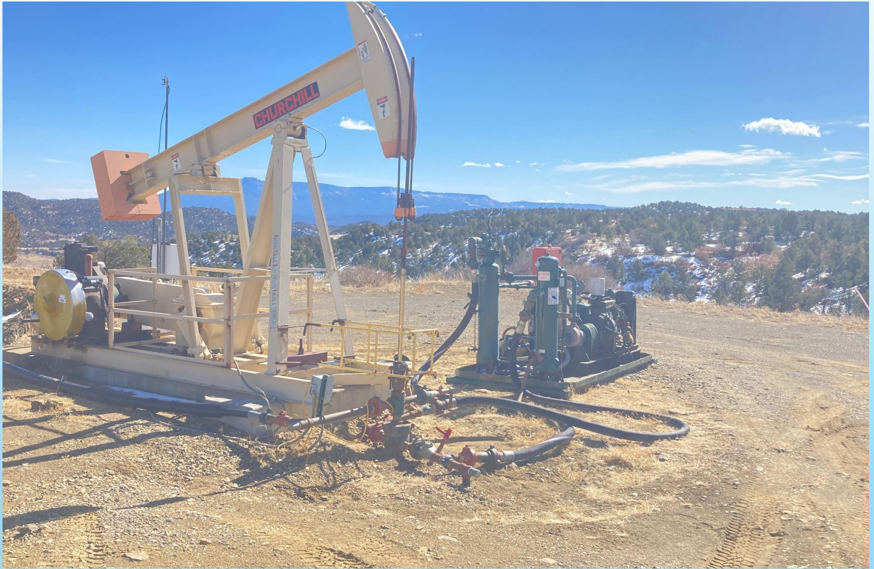
PHOTO 3: ORIGINAL WELLHEAD AND EQUIPMENT
