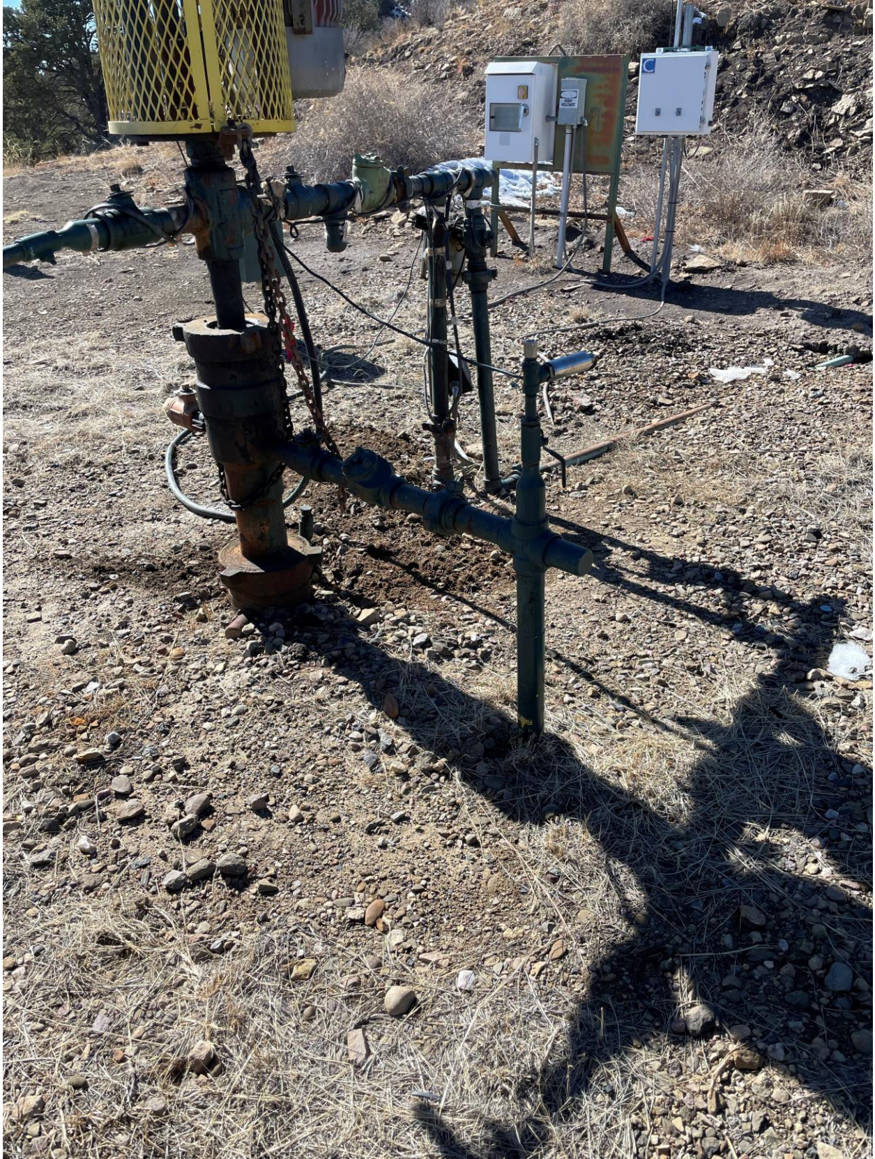
Removed unused equipment to comply with Rule 606
