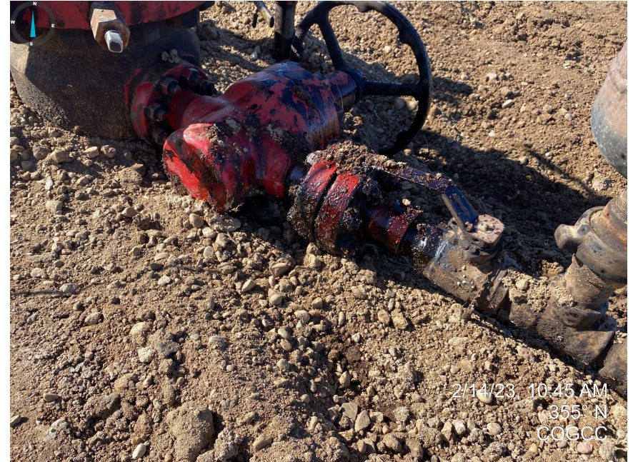
Photos 13 & 14. Close up photos near the wellhead and pump jack. Crude oil was observed from the stockpiled material leading to the well head; presence of crude oil was observed on piping as well.
