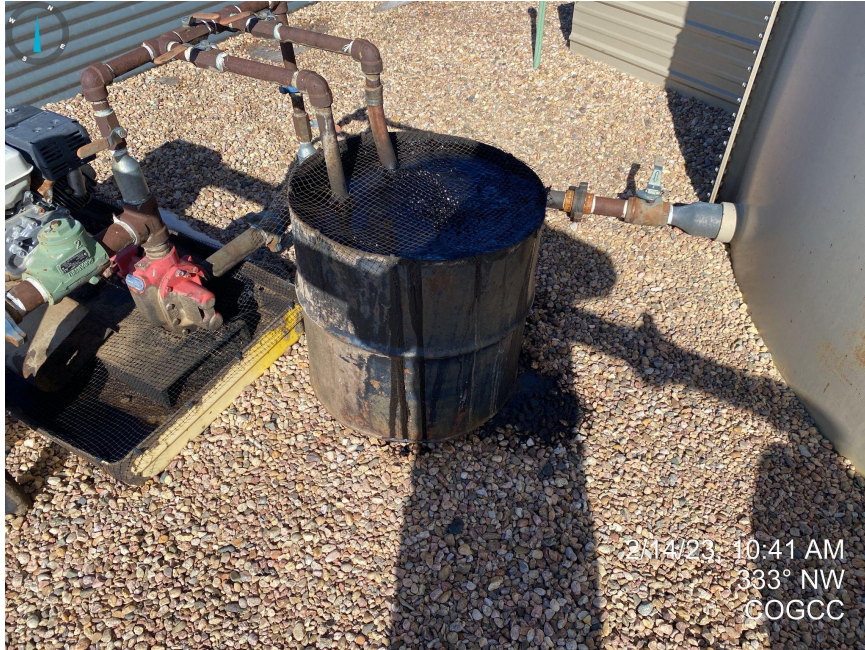
Photos 1 & 2. Facing northwest from inside of the tank battery containment. Photos illustrates an apparent leak originating from bucket/drum and staining the soil underneath.
