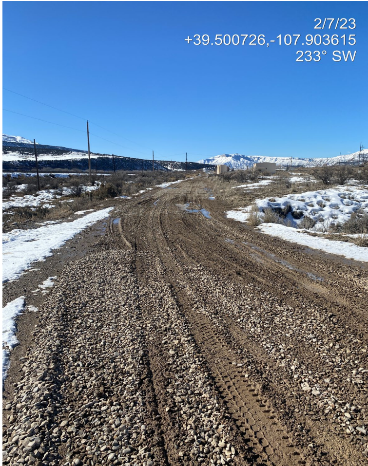
Photo 1. Photos show gravel has been added to the pad surface and access road.
