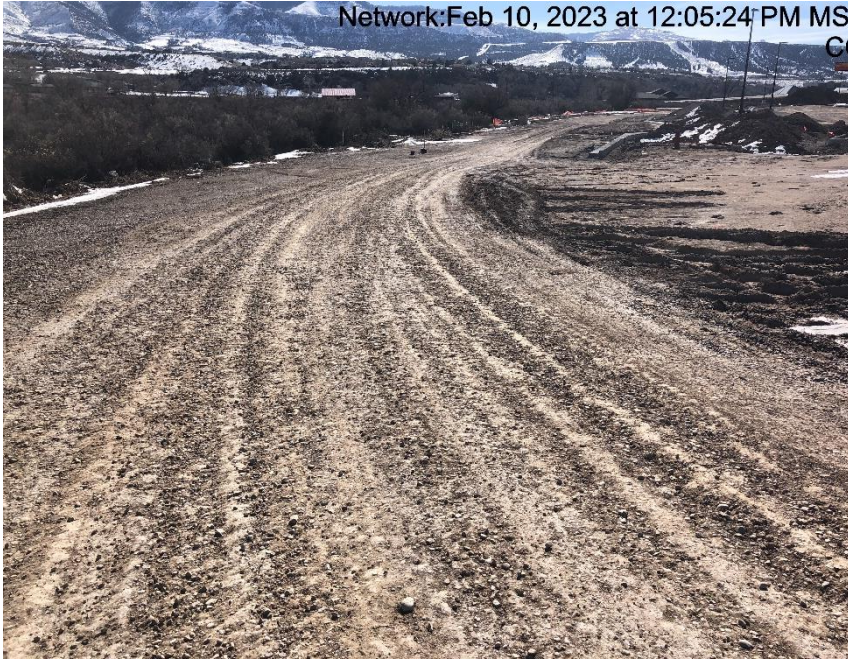
Photo #8979 Insufficient tracking BMP at entrance to location.
