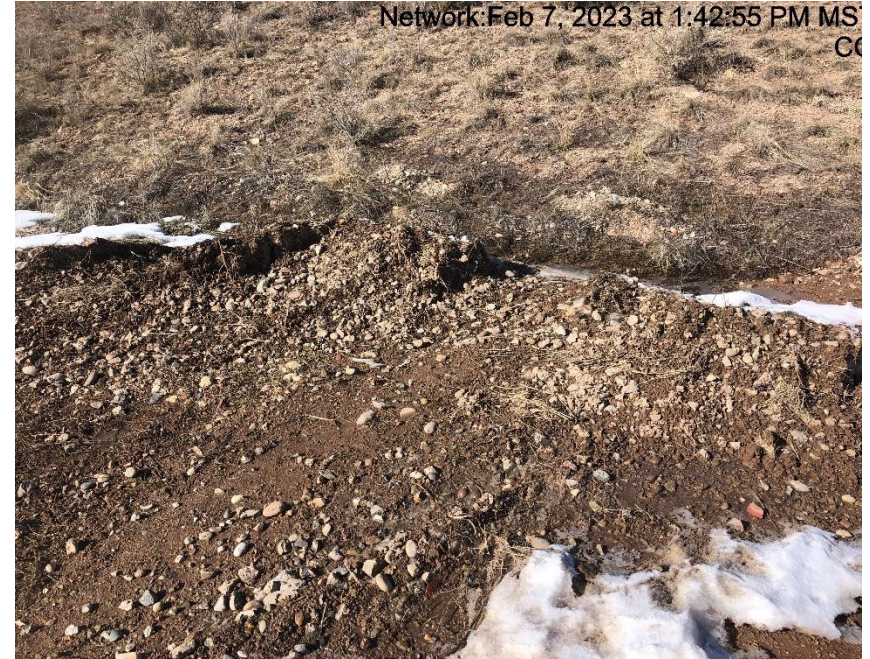
Photo #8937 Sediment has been transported into ditch.
