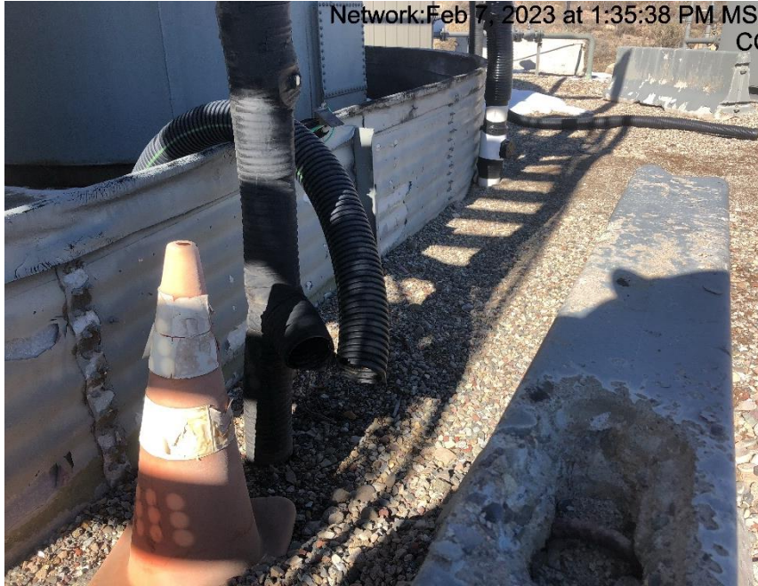
Photo #8925 Flow line heating insulation open ended.
