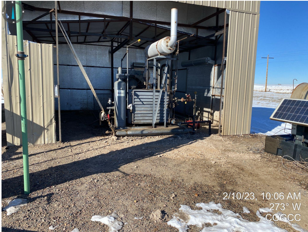
Photo 3. Facing west at compressor station. Photo illustrates that no wildlife protection devices (e.g. snow fence or similar) were installed when the antifreeze spill was observed during this inspection. Per 02/10/2023 phone call, Operator stated that they installed and took down snow fence after the antifreeze spill was cleaned up the first time (~01/24/2023). Operator will now have to reinstall wildlife protection device until spill is cleaned up.
