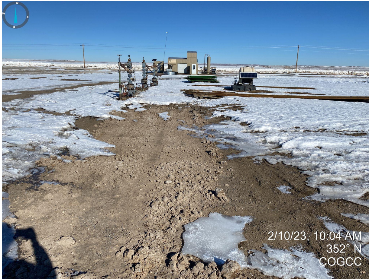
Photo 2. Facing north near the wellhead. The operator has removed the leaking tank from location and cleaned the stained soil. The other equipment pictured will be reinstalled after a nearby well is fracked, per 02/10/2023 phone call with Operator.
