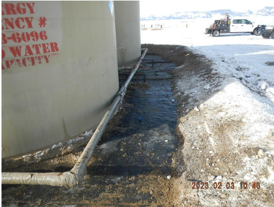
Photo 4. Photo taken from the NE corner of the tank battery. Crews have removed ice and pea gravel from on top of the secondary containment liner. Multiple tears are noted in the liner.
