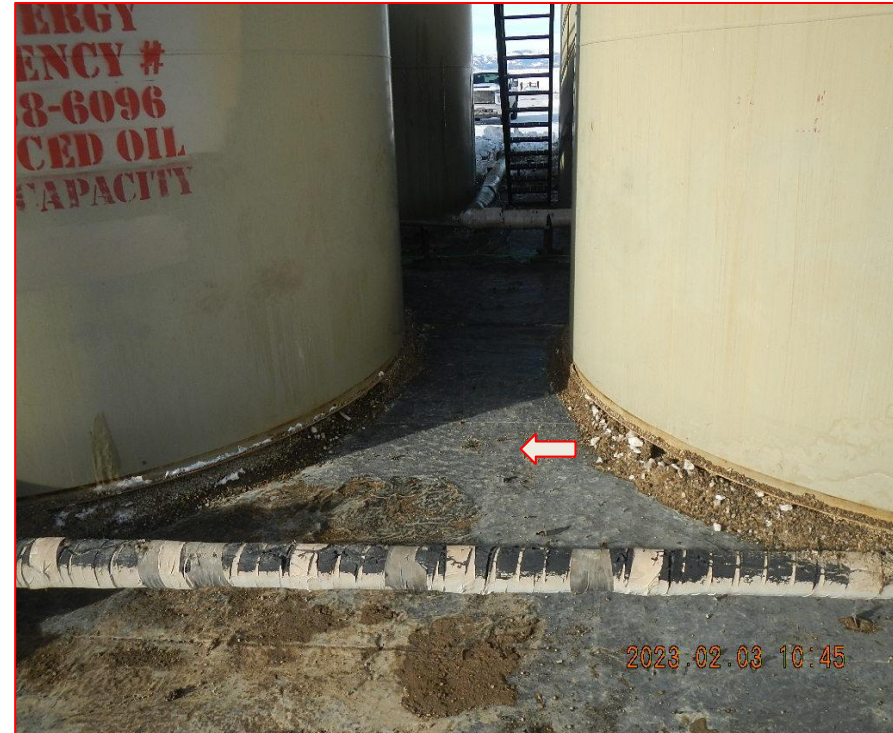
Photo 3. Photo taken from the east side of the tank battery. Crews have removed ice and pea gravel from on top of the secondary containment liner. Multiple tears are noted in the liner.
