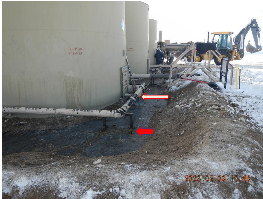
Photo 2. Photo taken from the NW corner of the tank battery. Crews have removed ice and pea gravel from on top of the secondary containment liner. Multiple tears are noted in the liner with shovels directly on the liner.
