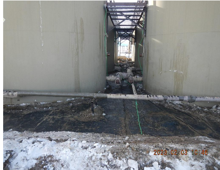
Photo 5. Photo taken from the north side of the tank battery. Crews have removed ice and pea gravel from on top of the secondary containment liner. Multiple tears are noted in the liner.
