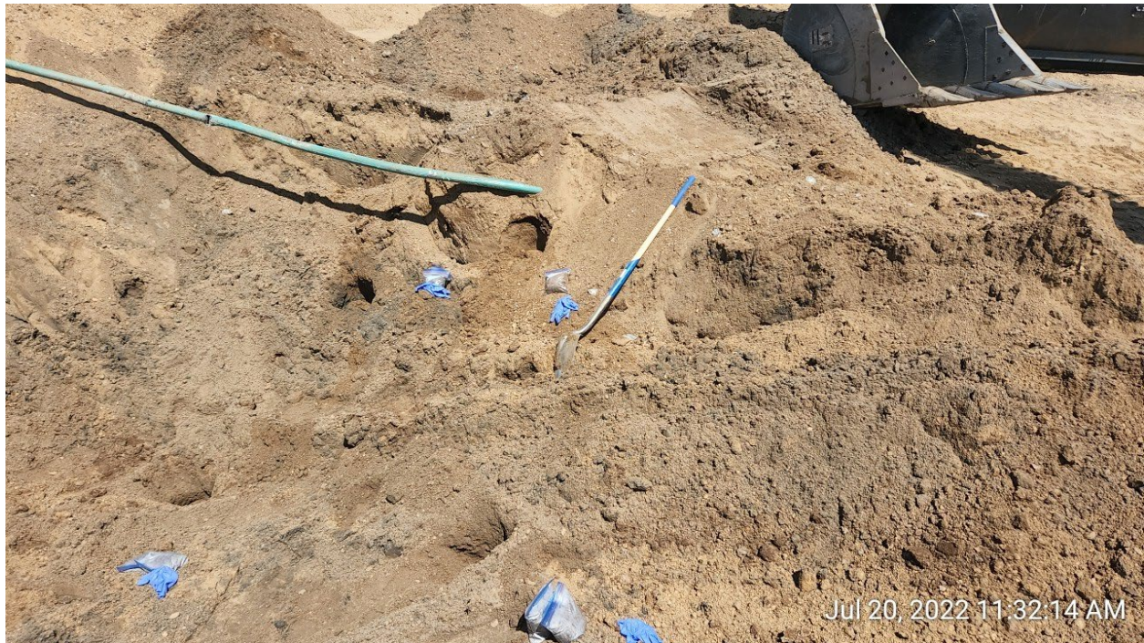
#3A – PTF-64N64W 32SENE – Dumplines – AST and PWV Tie-in - NDL02@2.0'– No Impacts Noted – PID 15.5ppm
