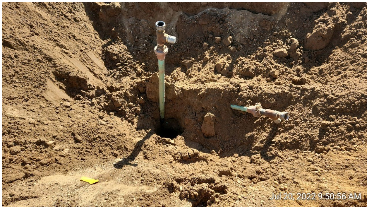
#3B – PTF-64N64W 32SENE – Dumplines – Separator Tie-in - NDL01@3.5'– No Impacts Noted – PID 1.7ppm
