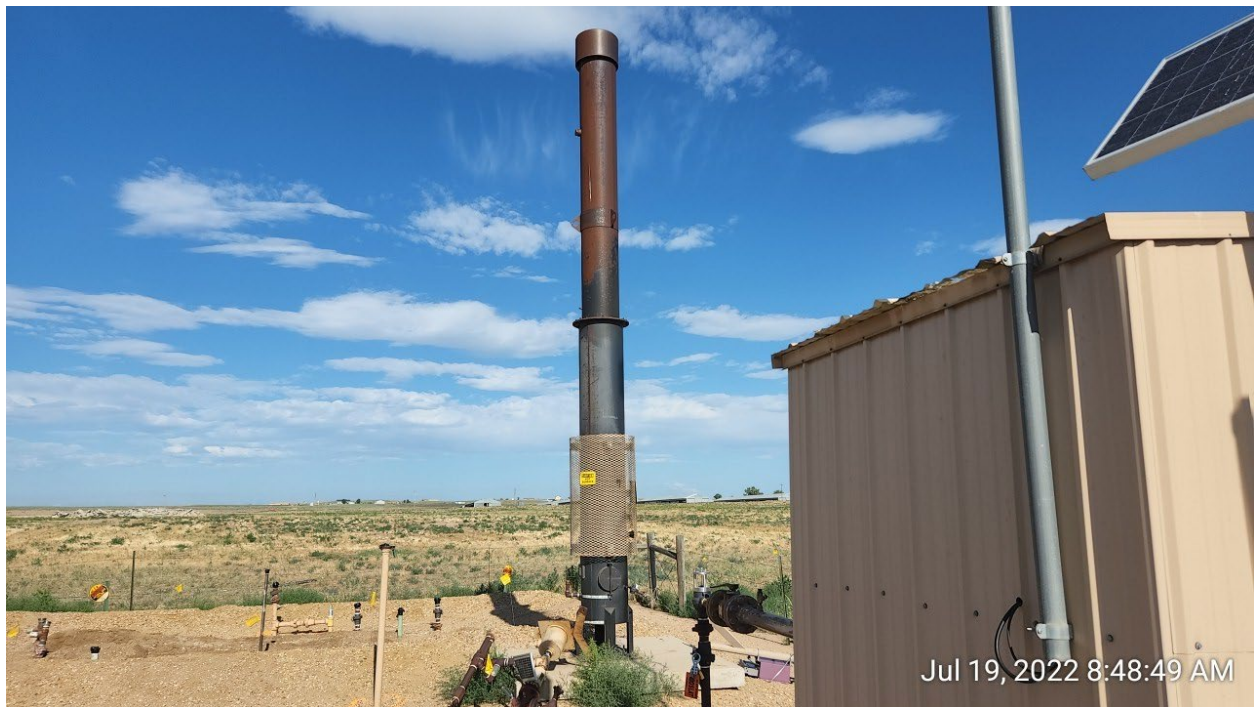
#5A – PTF-64N64W 32SENE – Combustion Unit – Good Condition – Minimal Corrosion – NECD01@6.0' – No Impacts Noted – PID 0.1ppm
