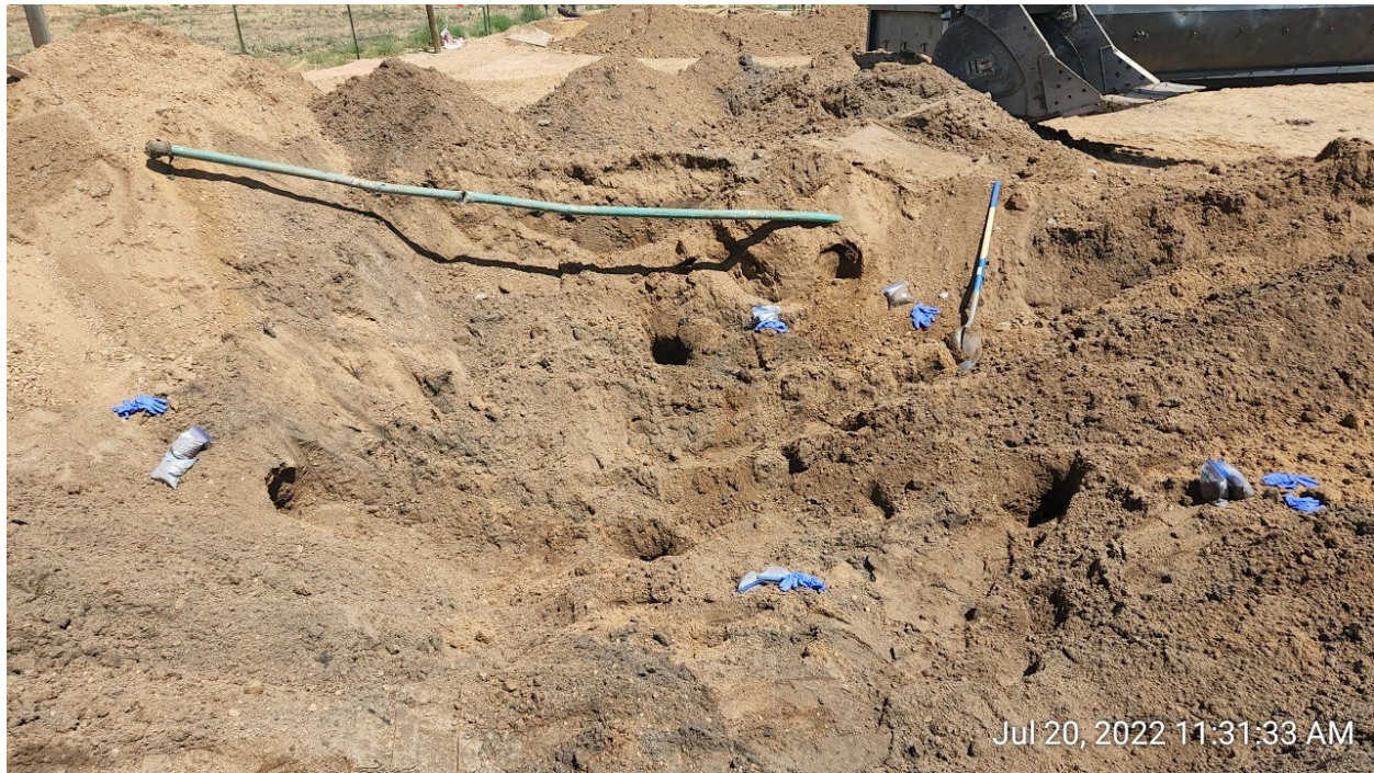
#2B – PTF-64N64W 32SENE – North Sidewall of Produced Water Vault Excavation – NPWVN01@4.0' – Staining and Odor Present – PID 803.9ppm – Sample Submitted for Lab Analysis
