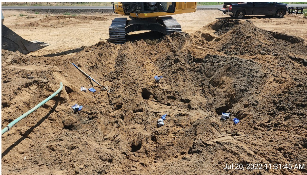
#2D – PTF-64N64W 32SENE – East Sidewall of Produced Water Vault Excavation – NPWVE01@4.0' – Staining and Odor Present – PID 371.5ppm – Sample Submitted for Lab Analysis
