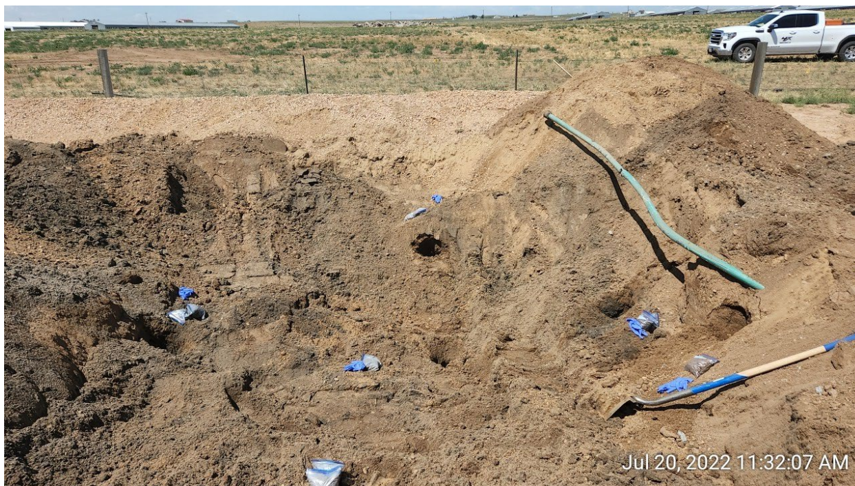
#2E – PTF-64N64W 32SENE – West Sidewall of Produced Water Vault Excavation – NPWVW01@4.0' – Staining and Odor Present – PID 466.4ppm – Sample Submitted for Lab Analysis
