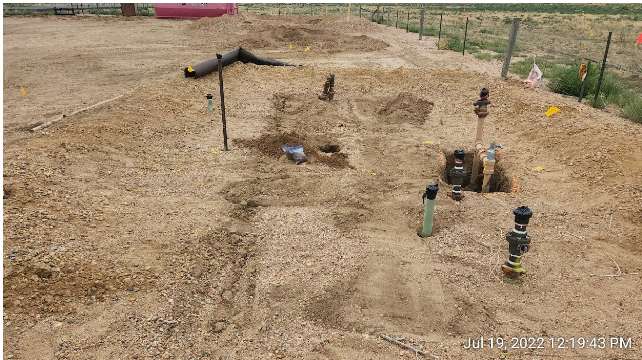
#4B – PTF-64N64W 32SENE – Separator – NSEP01@6.0' – No Impacts Noted – PID 1.0ppm
