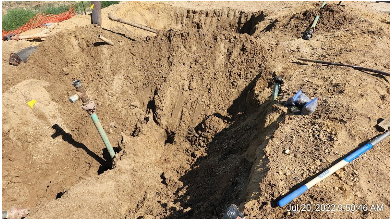
#4C – PTF-64N64W 32SENE – Separator – NSEP02@3.5' – No Impacts Noted – PID 1.0ppm – Sample Submitted for Lab Analysis
