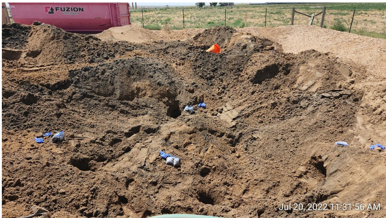
#2C – PTF-64N64W 32SENE – South Sidewall of Produced Water Vault Excavation – NPWVS01@4.0' – Staining and Odor Present – PID 992.3ppm – Sample Submitted for Lab Analysis
