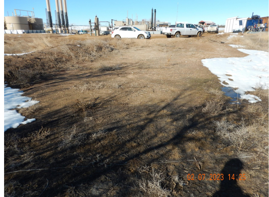
Photo 6. Photo taken from a portion of the flowline, facing North. Photo illustrates bare soil with no vegetation to stabilize the area. Erosion control blankets were previously used within the flowline area but are no longer functioning.
