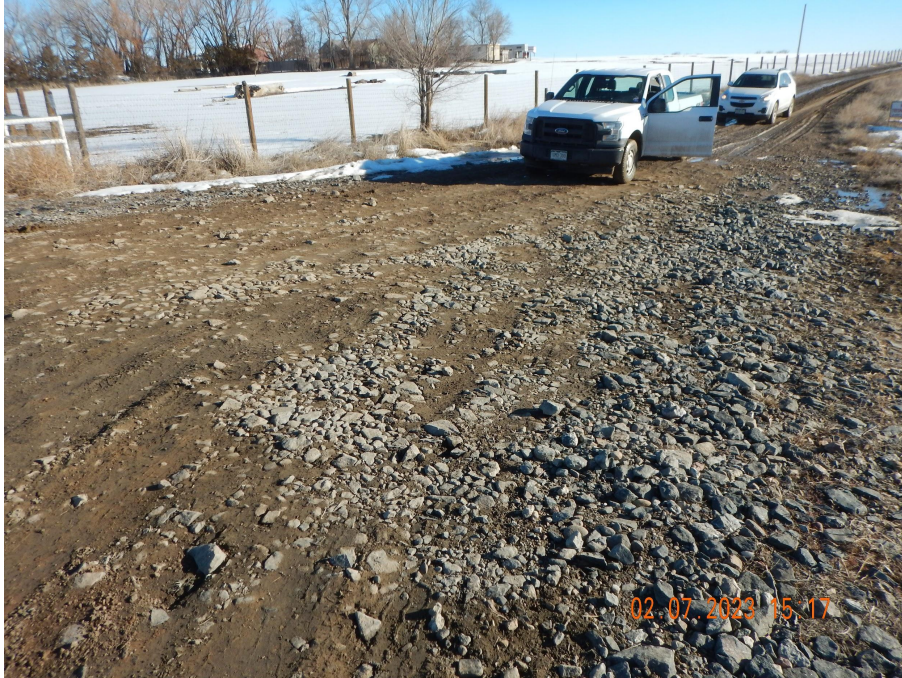
Photo 7. Photo taken from the entrance of location, facing South. Photo illustrates the vehicle tracking device BMP is in need of maintenance. At the time of this inspection, there was no track out observed.
