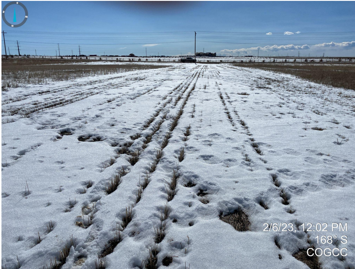
Photo 2. Facing south from the former access road. See comments in Photo 1.
