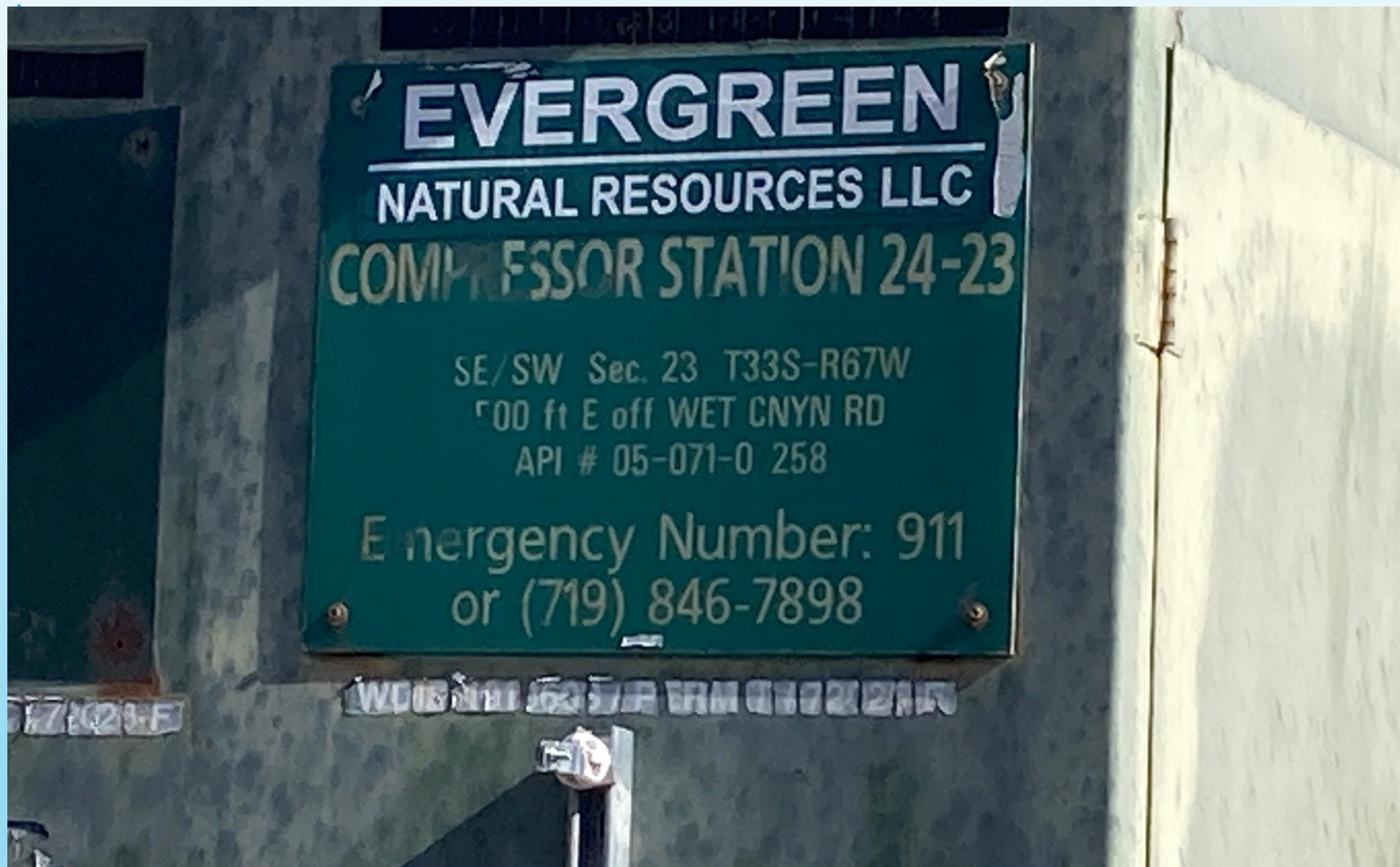
PHOTO 1: WELL SIGN/ API# IS FADED AND NEEDS REPOSTED. Install sign to comply with Rule 605.a. CA DATE 3/7/2023.
