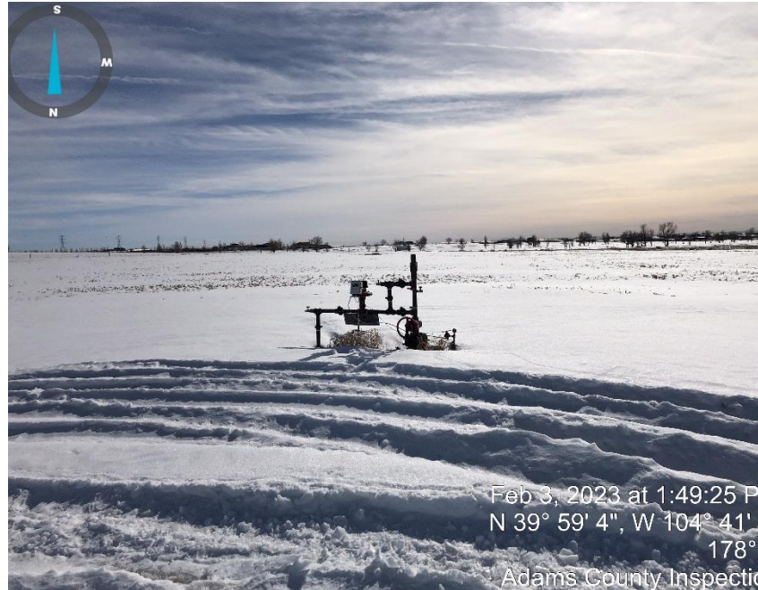
Photo# 3 Well Head.
