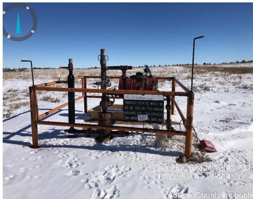
Photo# 3 Well Head.
