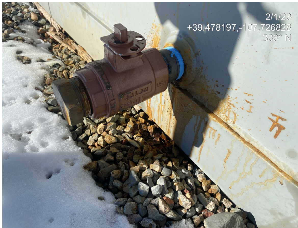
Photo 2. Photo show staining at the separator for well API #045-07462.
