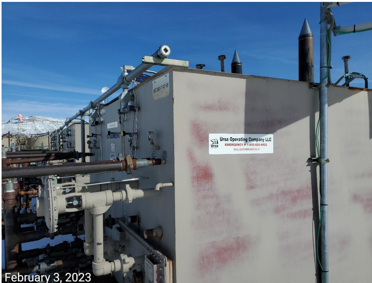
Photo 3: Photo example showing incorrect label information observed on the Separator equipment.
