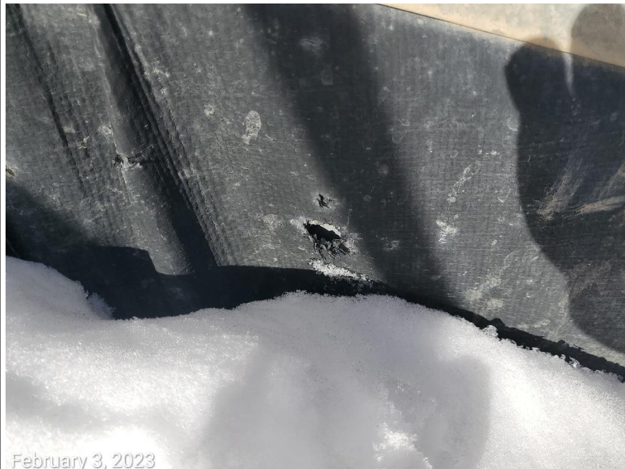
Photo 1: Photos examples showing various holes/tears observed at the tank battery's secondary containment.
