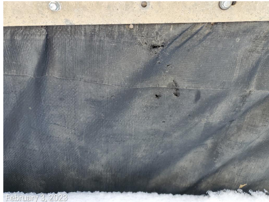
Photo 1: Photos examples showing various holes/tears observed at the tank battery's secondary containment.
