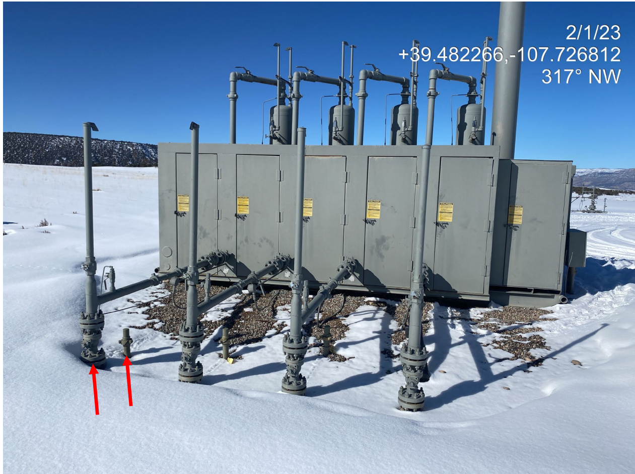
Photo 2. Photo shows two (2) risers which appear to be associated with a plugged and abandoned well and decommissioned flowline.
