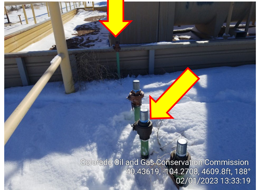
Photo 12 – Unmarked Riser – Middle Riser and 1" at Berm
