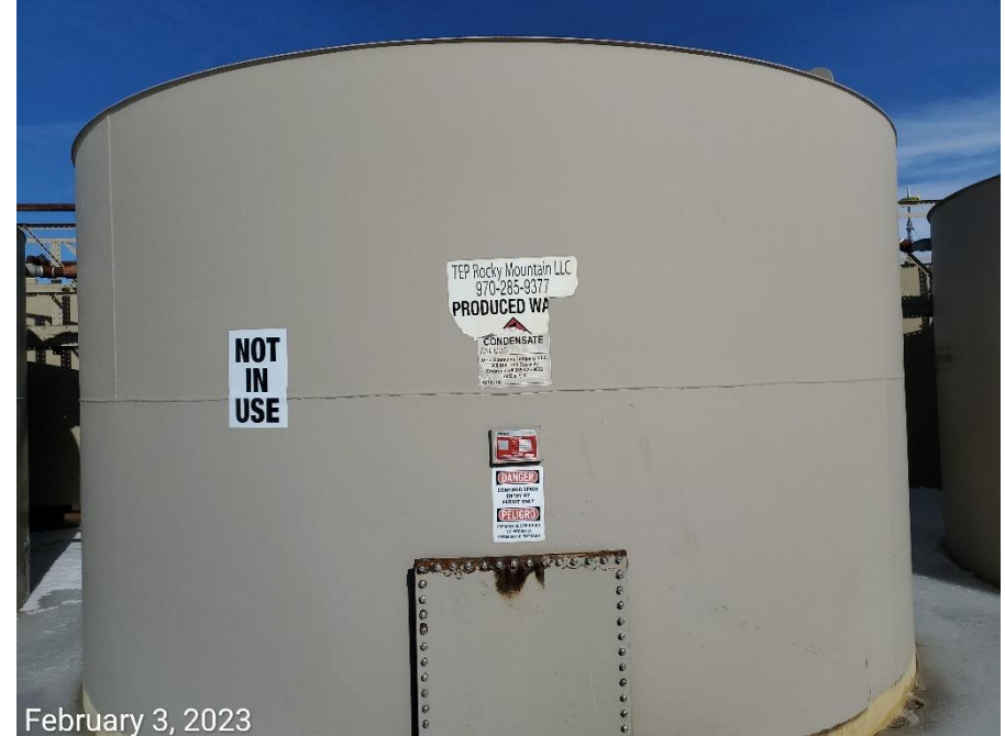
Photo 6: Photos show tank signage/labeling is either missing, or inaccurate.
