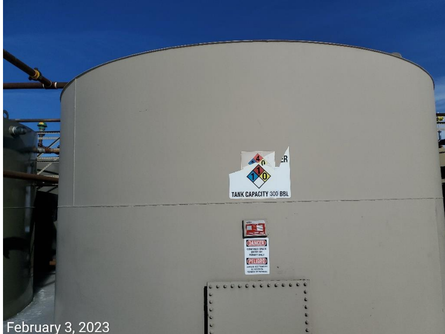
Photo 6: Photos show tank signage/labeling is either missing, or inaccurate.
