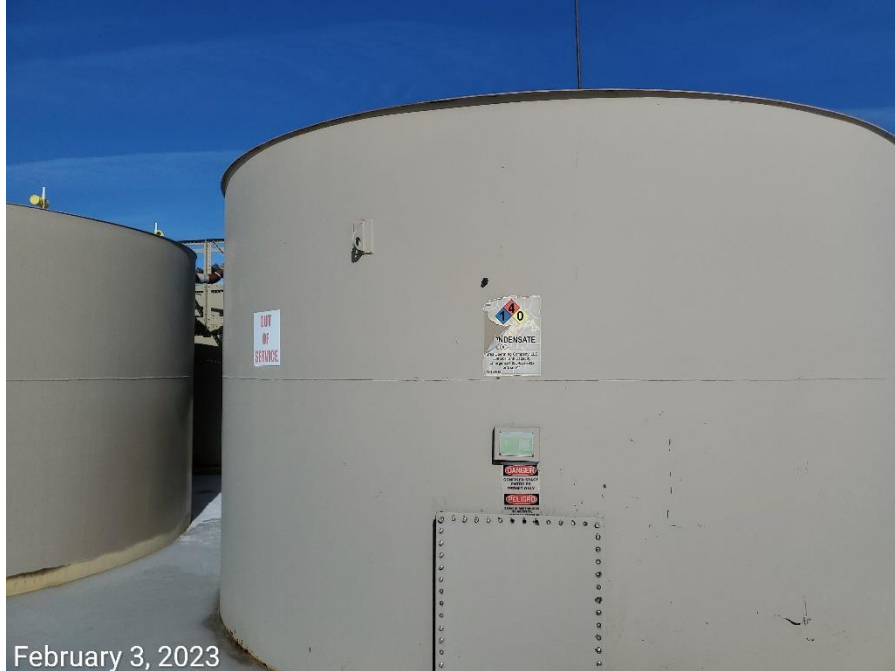
Photo 7: Photos show tank signage/labeling is either missing, or inaccurate.
