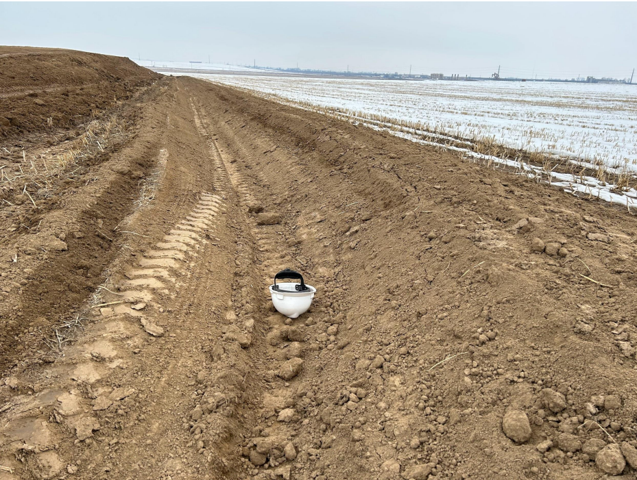
Photo 3. Photo taken from the western perimeter of location, facing south. Photo illustrates a berm and ditch BMP installed around the perimeter of the location.
