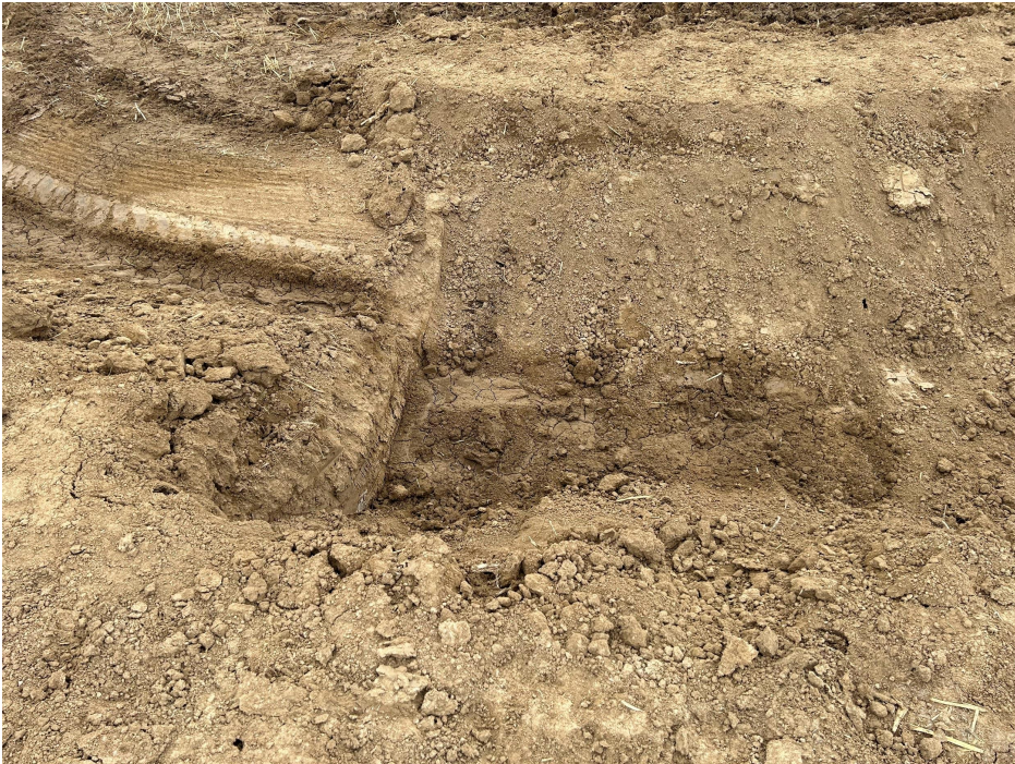
Photo 5. Photo taken of a sediment trap on location. . Photo illustrates the BMP is under construction but appears to be undersized to accommodate the size of the disturbance.
