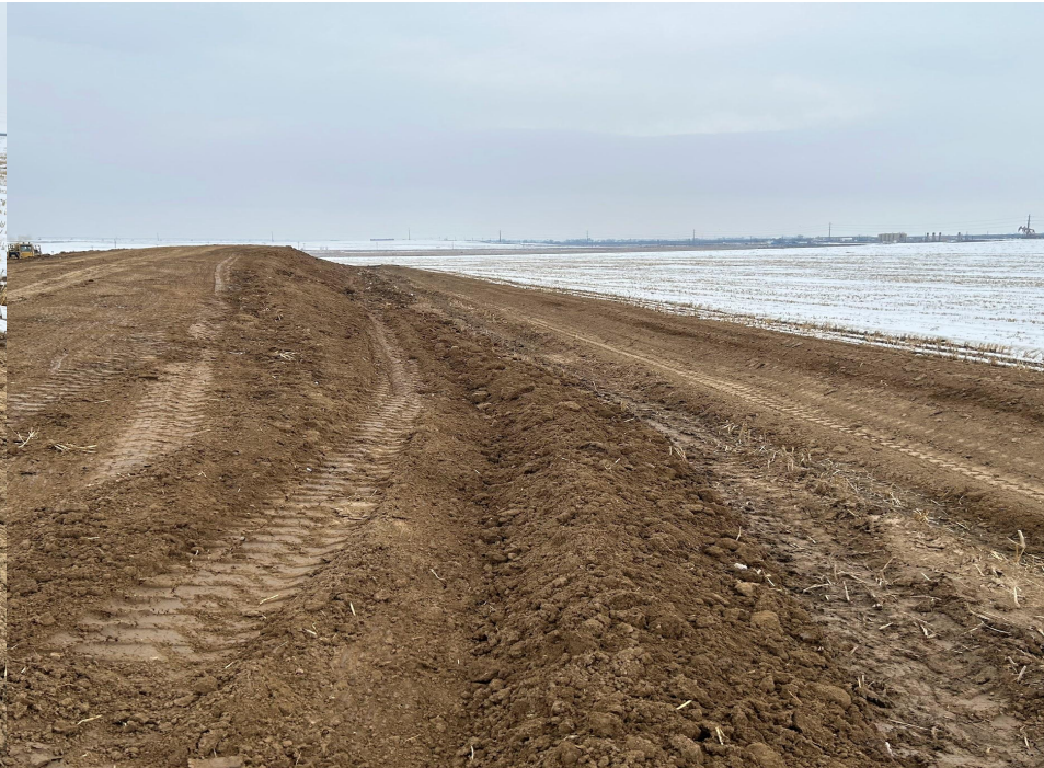
Photo 4. Photo taken from the topsoil stockpile on location. Stockpile is unconsolidated and shall be stabilized, per rule 1002c.
