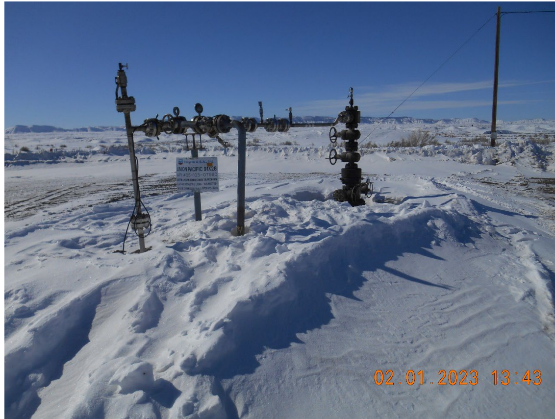
Injection Wellhead
