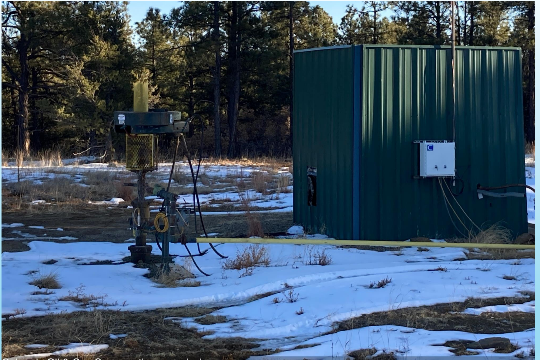
PHOTO 3: ORIG. WELLHEAD AND EQUIPMENT
