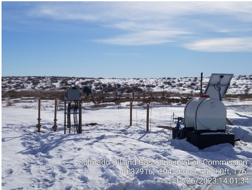
Photo 5 – Gas Lift Injection Meters
