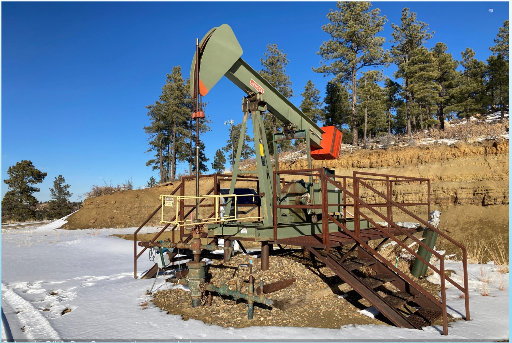
PHOTO 3: WELLHEAD AND EQUIPMENT
