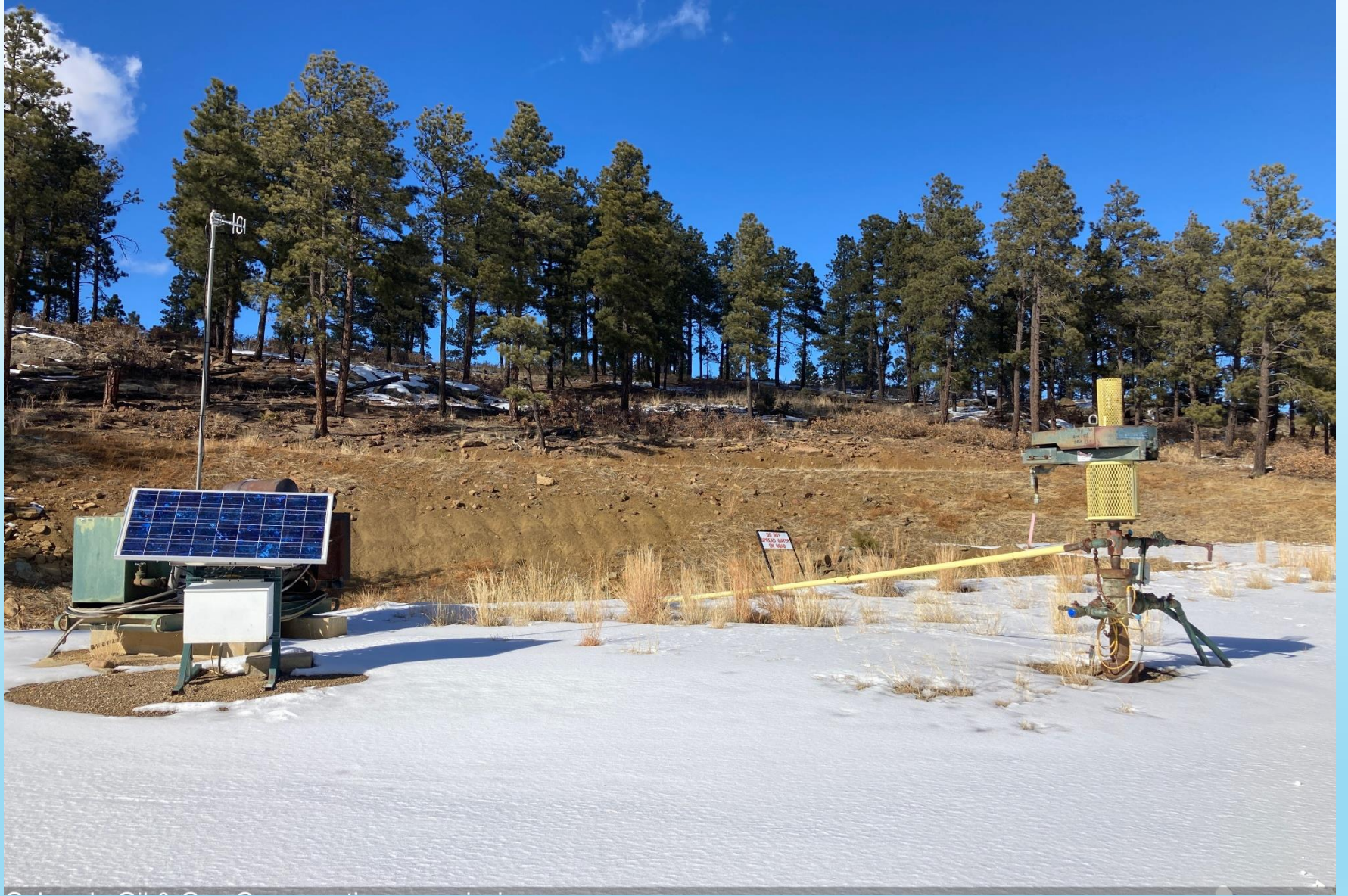
PHOTO 3: WELLHEAD AND EQUIPMENT
