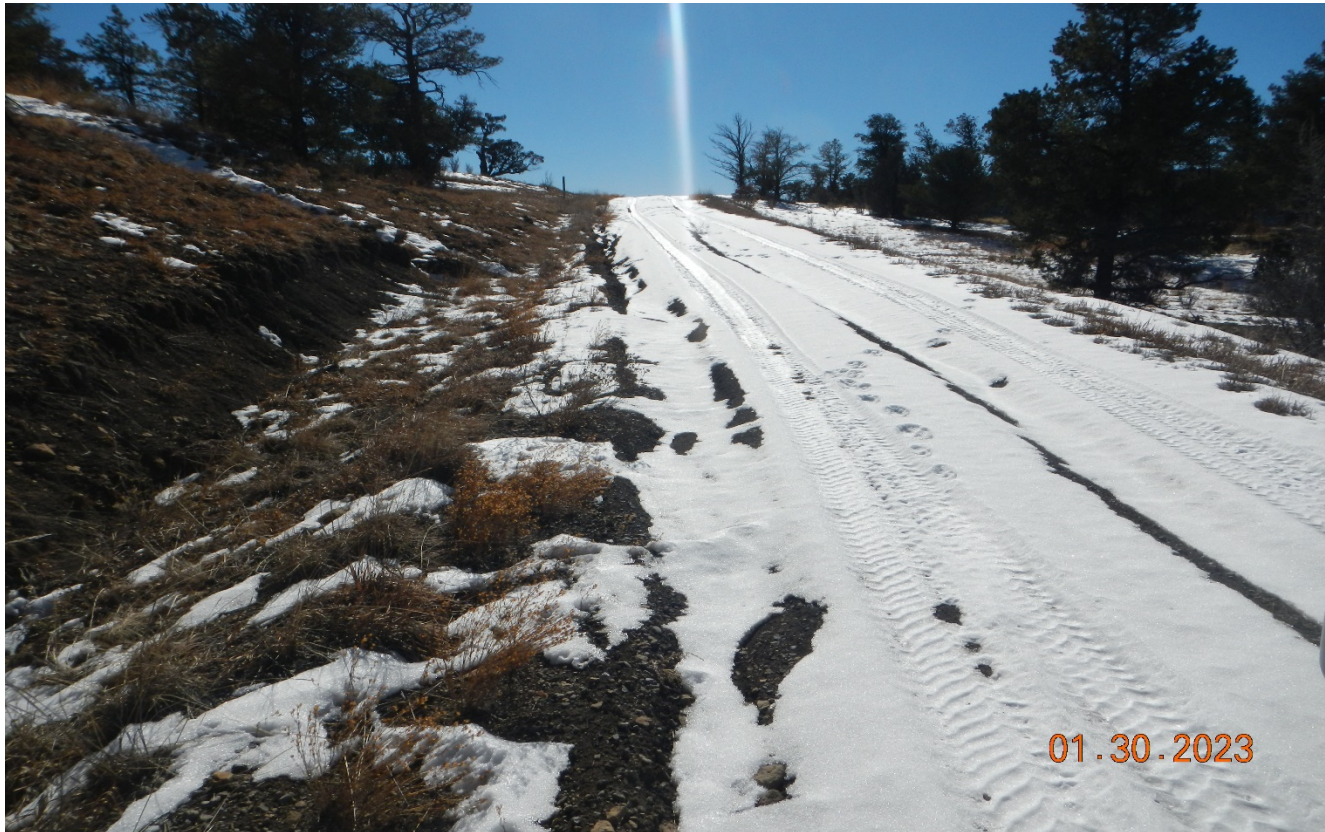
Photo 1. Facing southeast along the access road. This area of the road may need grading due to signs of vehicle rutting.
