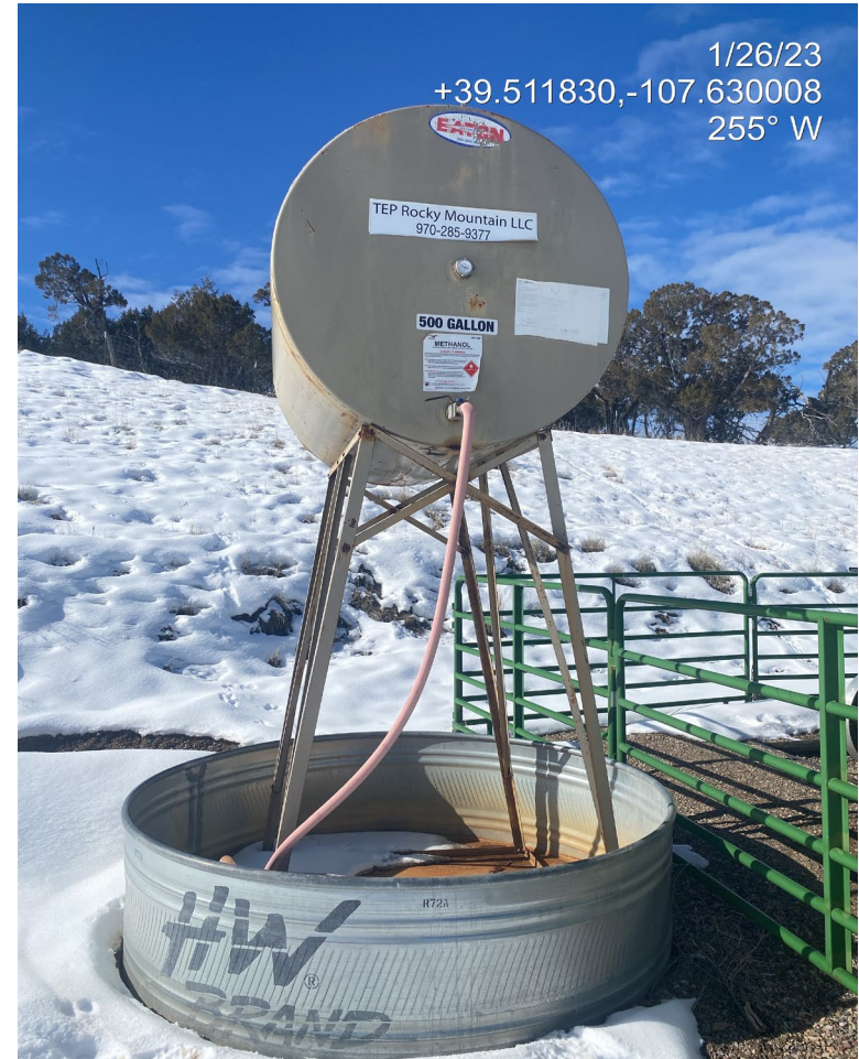
Photo 2. Photos show a cap not installed on a tank drain line (left) and wildlife protection BMPs absent on a secondary containment stock tank (right).
