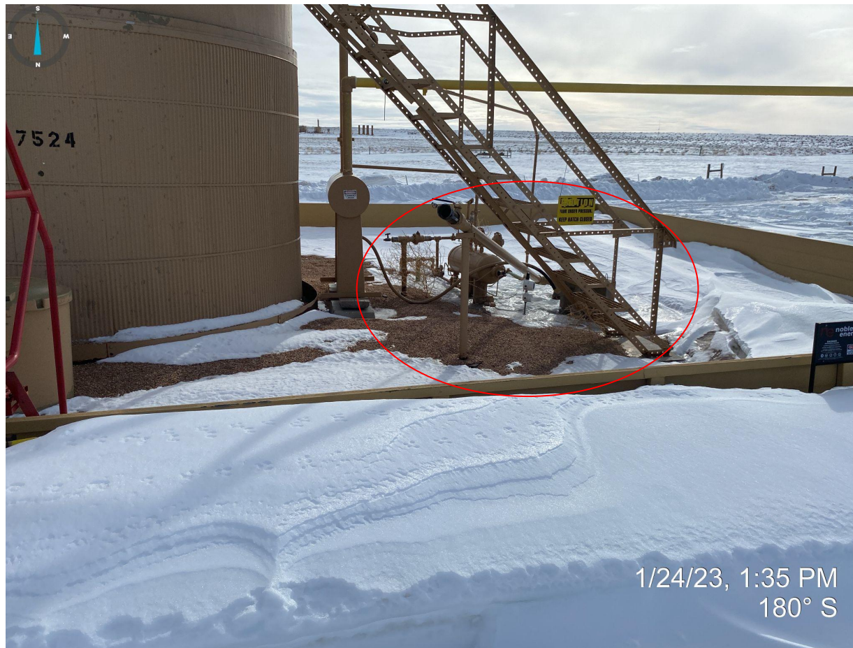
Photo 1. Facing south at the tank battery; undesirable vegetation (now considered debris) observed next to equipment. This should be disposed of as it presents a fire hazard.
