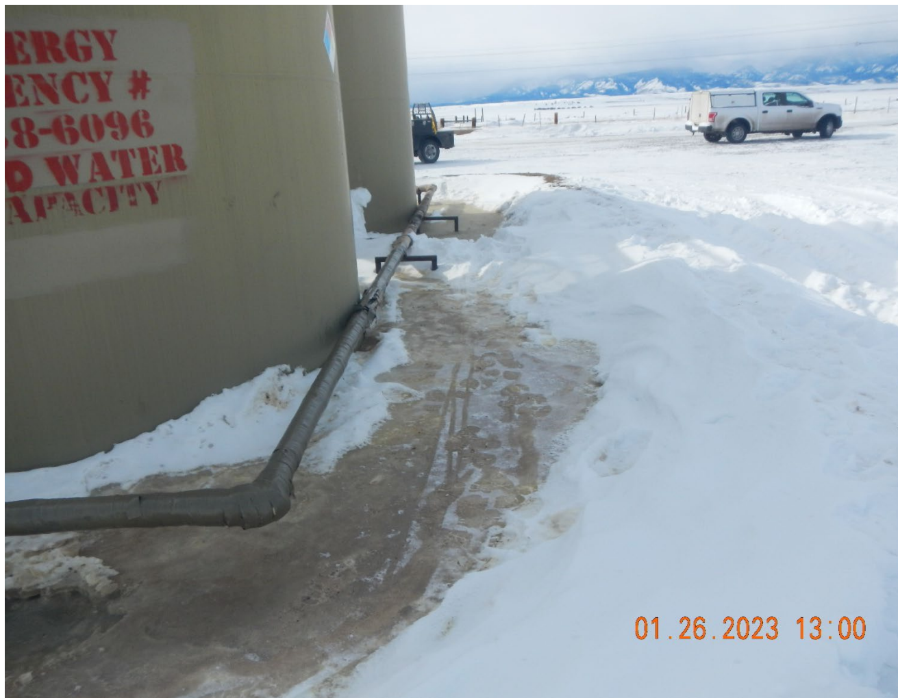
Photo #7 north side of tank battery. Frozen produced water.
