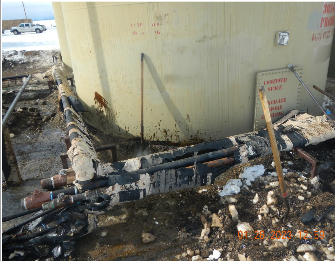
Photo #4 The Valve at left of photo is the valve that froze and released the produced water. Photos 1-4 show the area were Ice was chipped by hand and loaded into a side dump for offsite disposal as E&P waste.
