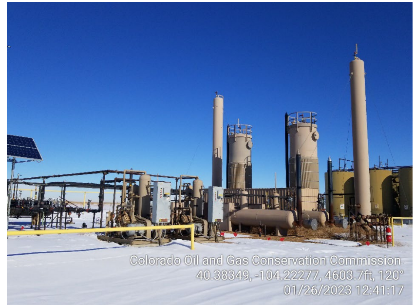
Photo 2 – VRUs, Separators, Treaters and VRTs
