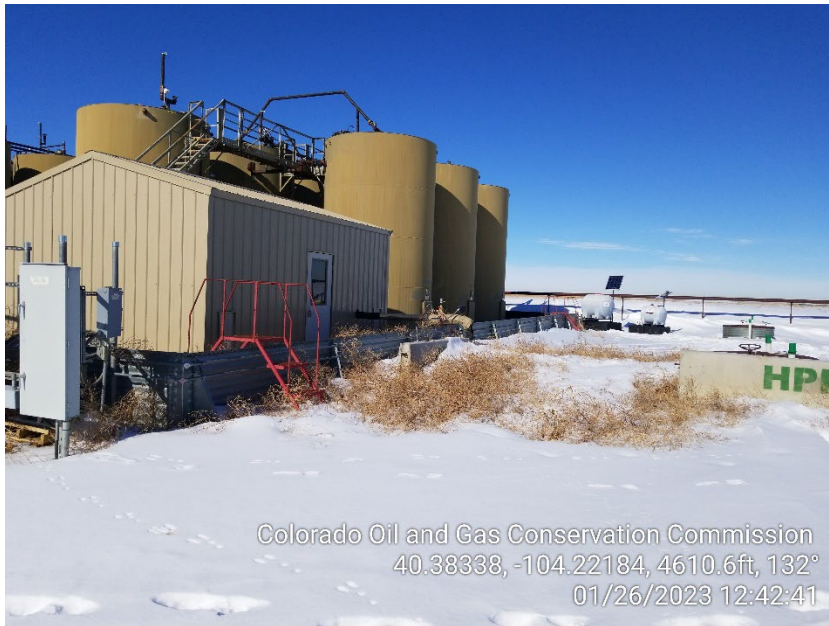
Photo 7 – Central Tank Battery and LACT – Tumbleweeds
