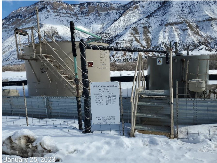
Photo 2: Tank battery. Photo on the right shows labeling at the larger tank is no longer legible.
