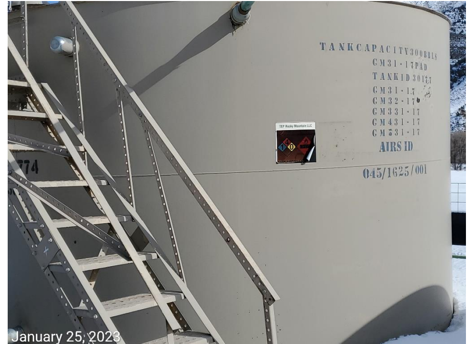
Photo 2: Tank battery. Photo on the right shows labeling at the larger tank is no longer legible.
