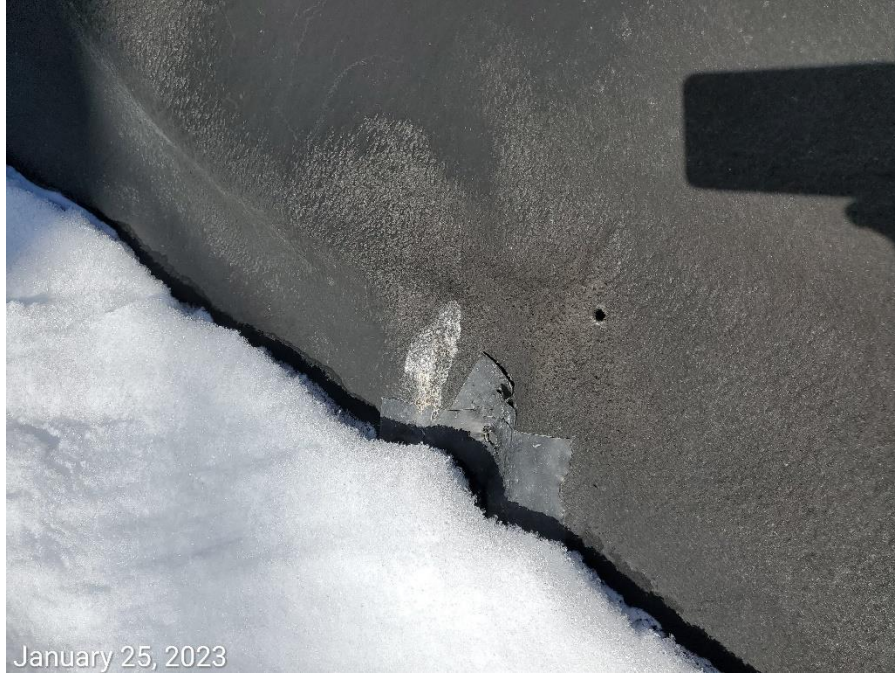
Photo 3: Photos examples showing various holes/tears observed within the secondary containment liner.
